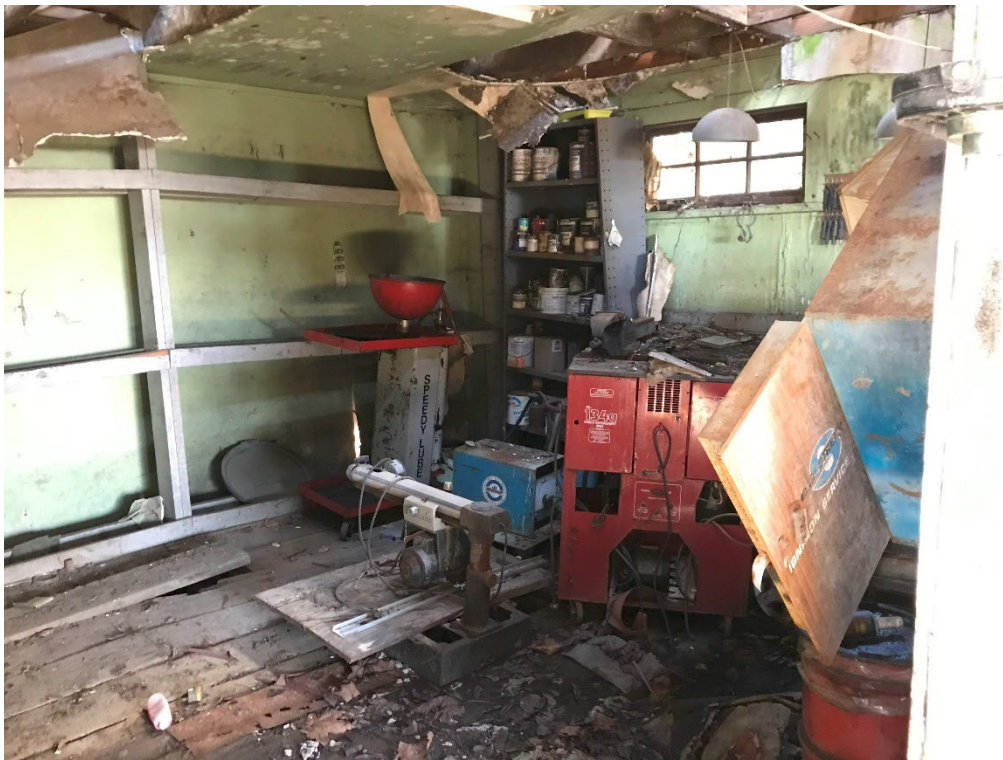
Photo 20: Miscellaneous storage within two-storey barn (old shop/office) at 240 Okotoks Road.
