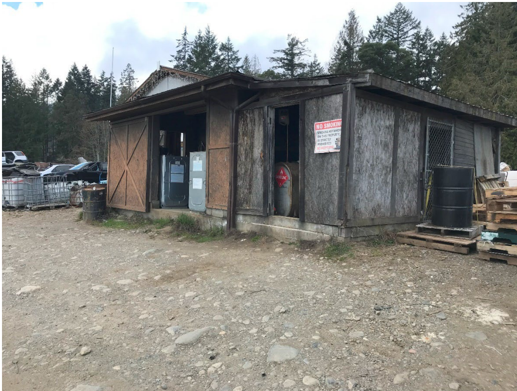
Photo 24: Oil shed building at 240 Okotoks Road.
