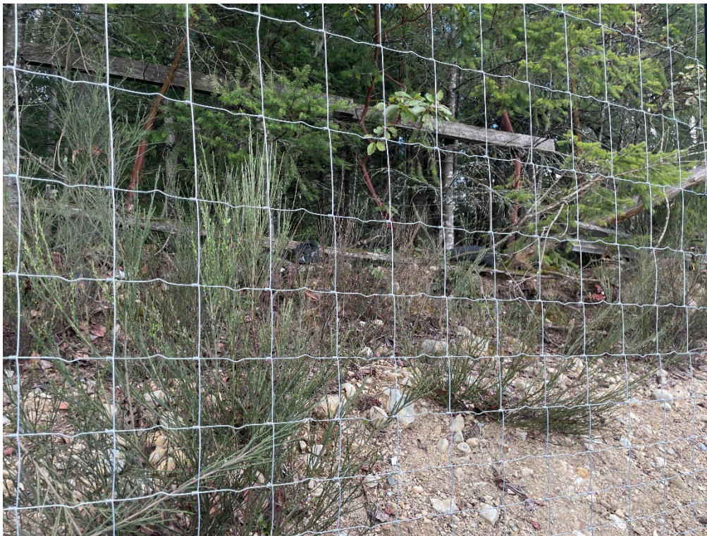
Photo 4: Post and page wire fence on the west property line of 240 Okotoks Road.
