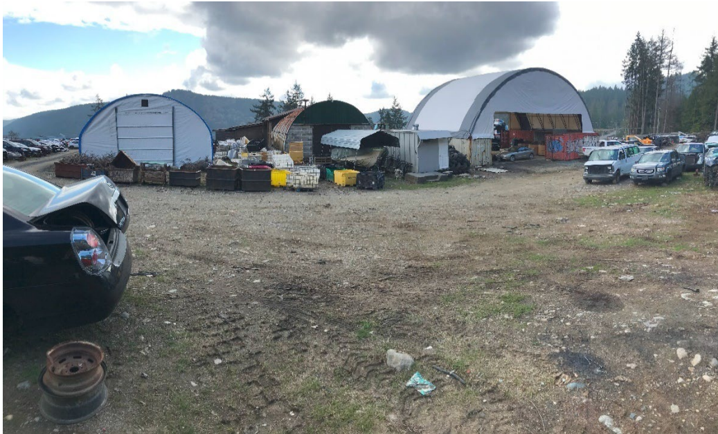
Photo 23: Concrete Block Dome, flanked by the Seacan Dome and Dome Tent at 240 Okotoks Road.
