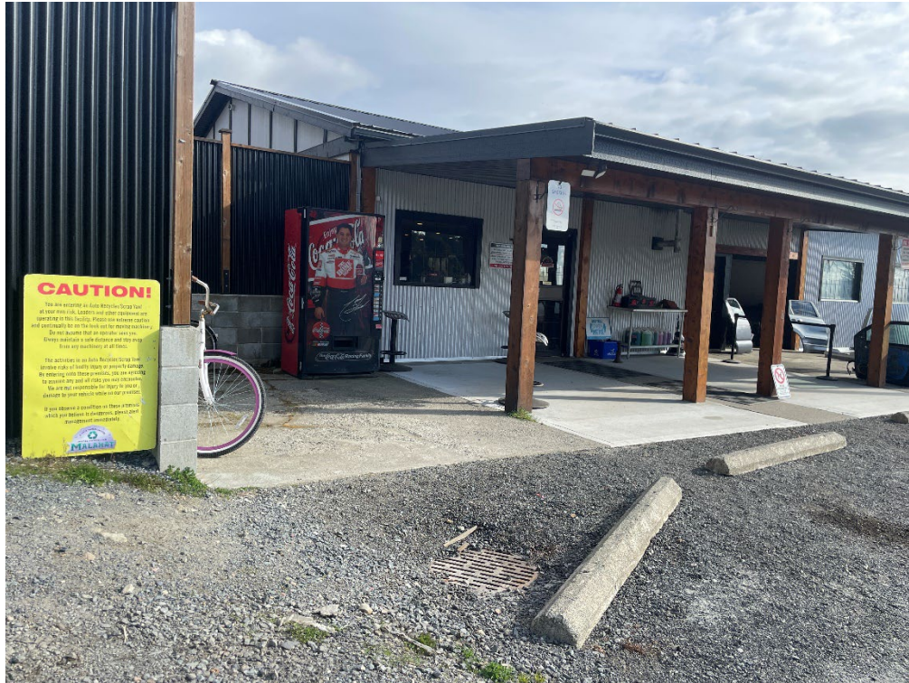
Photo 5: Main office building at 240 Okotoks Road.
