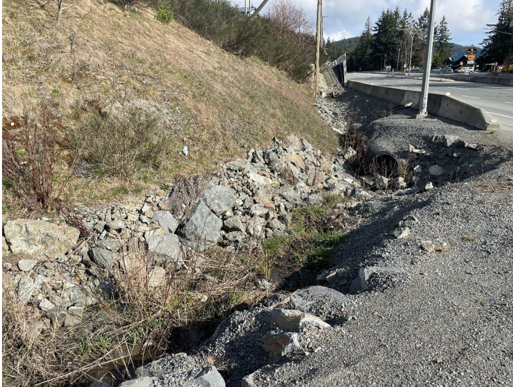
Photo 17: Drainage spillway of the main office roof leaders at 240 Okotoks Road.
