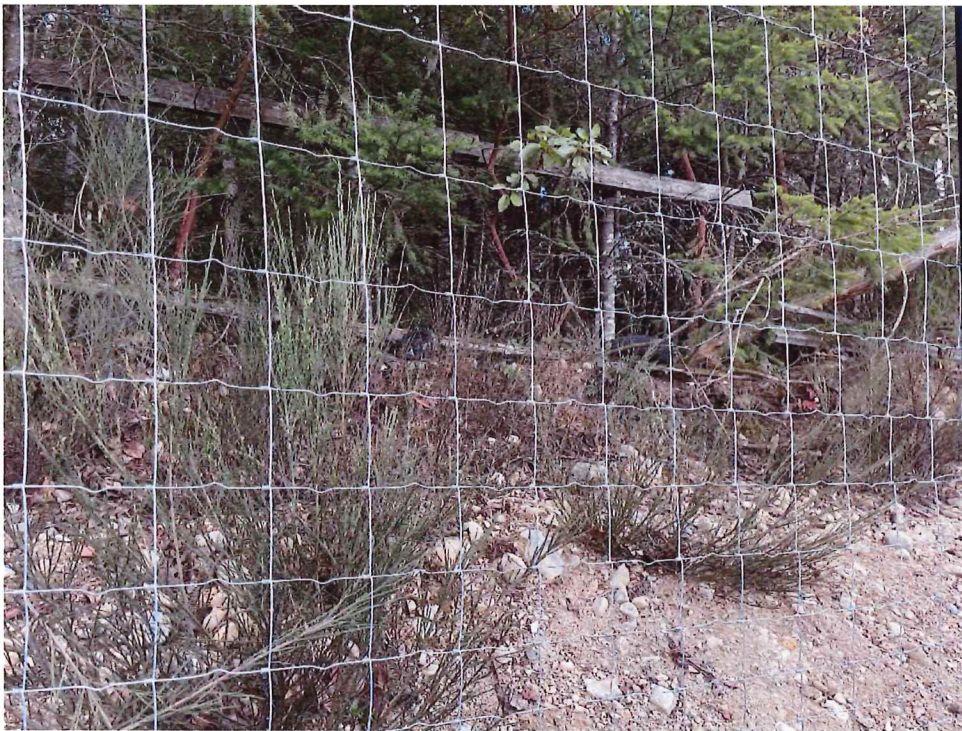
Photo 4: Post and rail wire fence on the west property line of 240 Okotoks Road.
