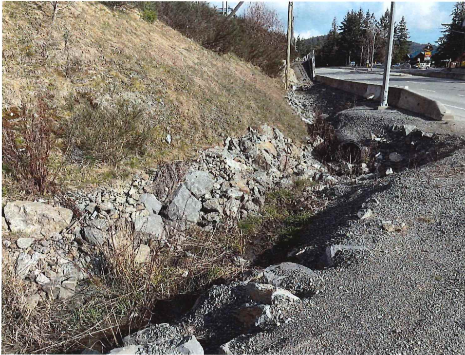
Photo 17: Drainage spillway of the main office roof leaders at 240 Okotoks Road.
