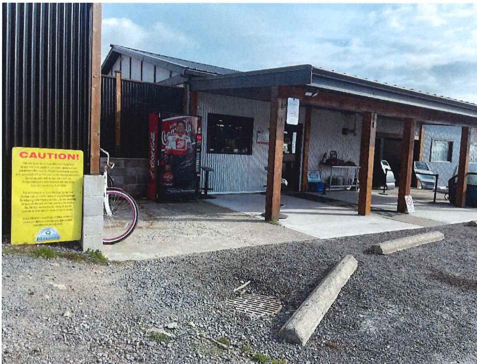
Photo 5: Main office building at 240 Okotoks Road.
