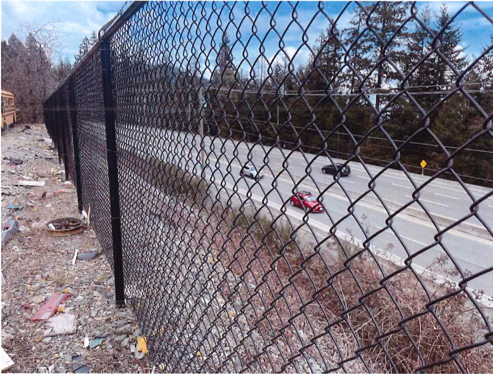
Photo 3: Typical chain link fence on east and south property line of 240 Okotoks Road.
