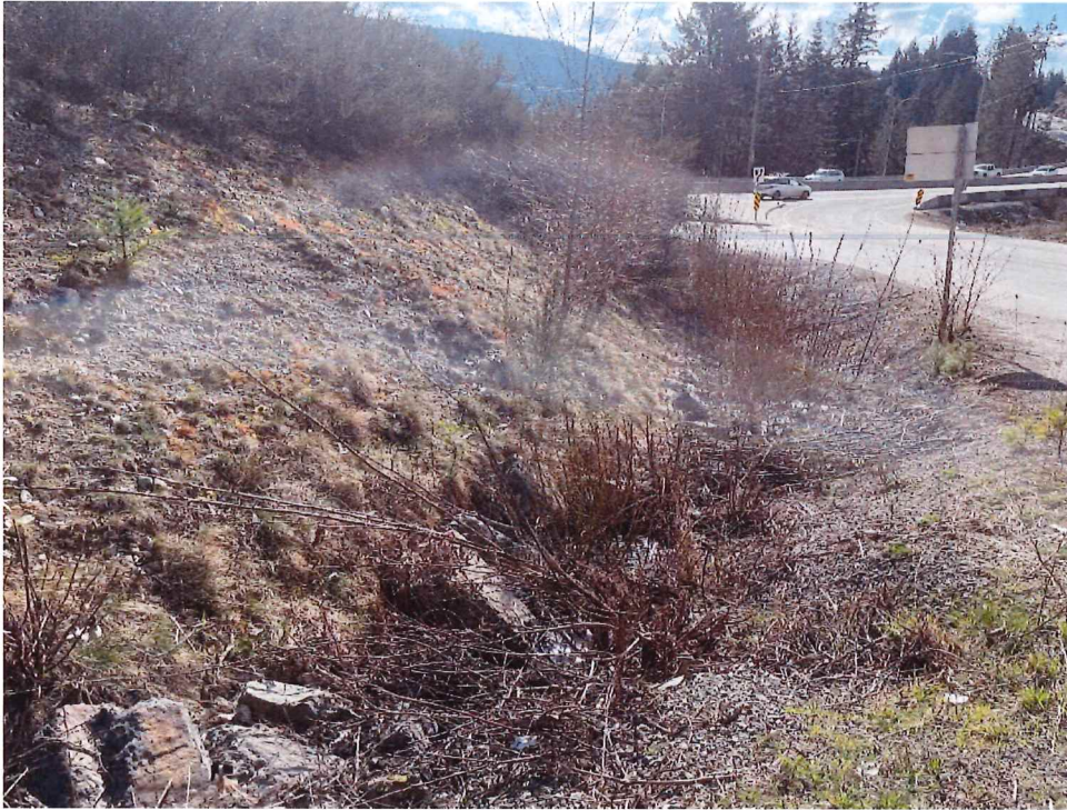
Photo 19: Drainage ditch for perimeter drain and parking lot of 240 Okotoks Road.
