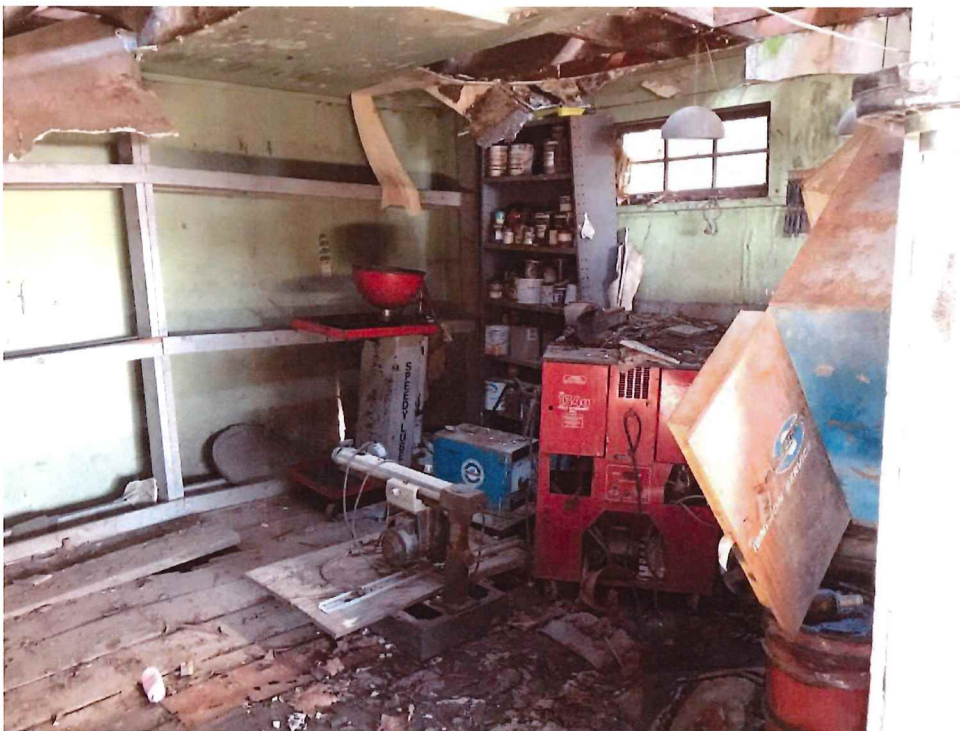
Photo 20: Miscellaneous storage within two-storey barn (old shop/office) at 240 Okotoks Road.
