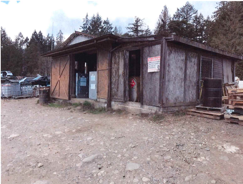
Photo 24: Oil shed building at 240 Okotoks Road.
