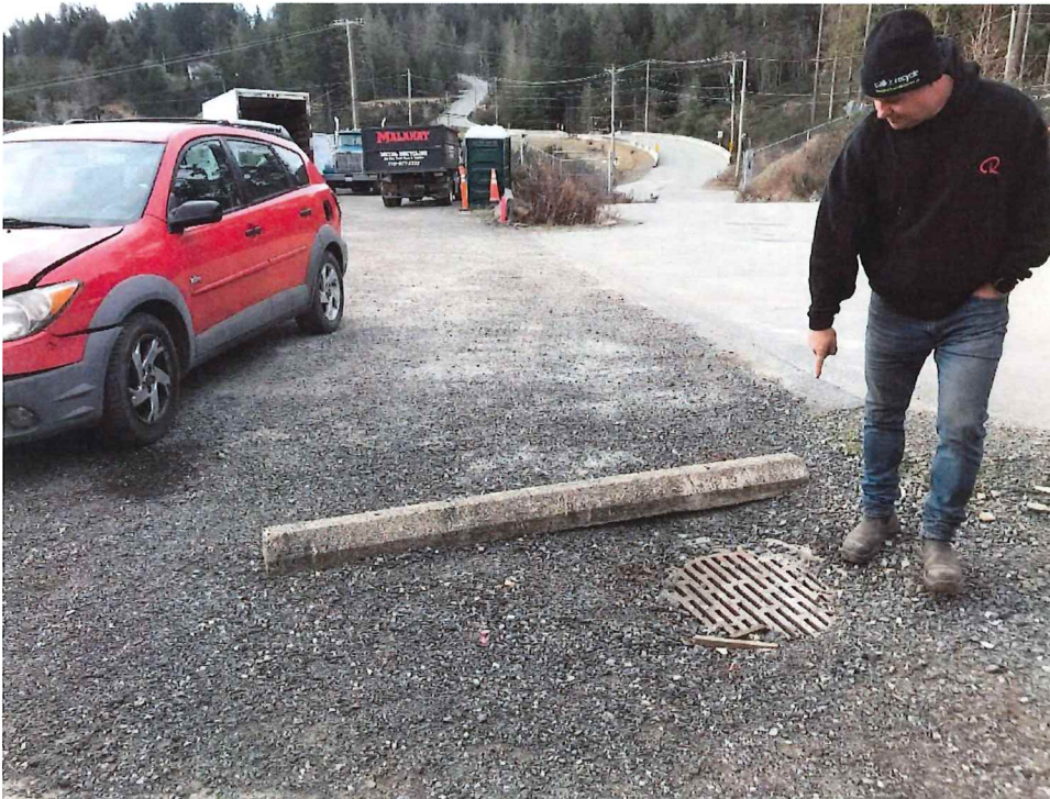
Photo 18: Slotted manhole cover in parking lot for overland flow and connected to the perimeter drain at 240 Okotoks Road.
