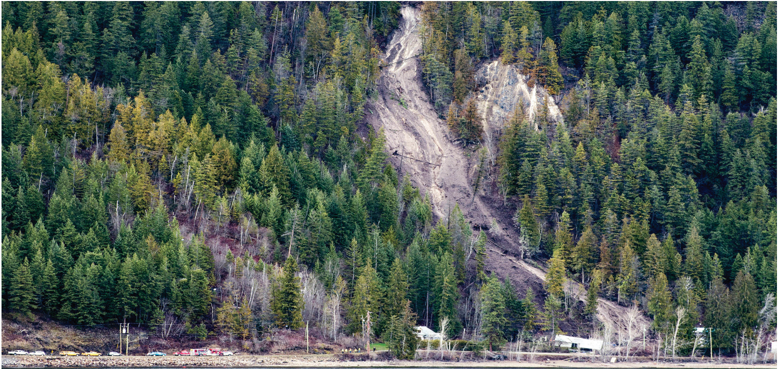
Image 2.4 Development at the toe-of-slope faces increased risk.
