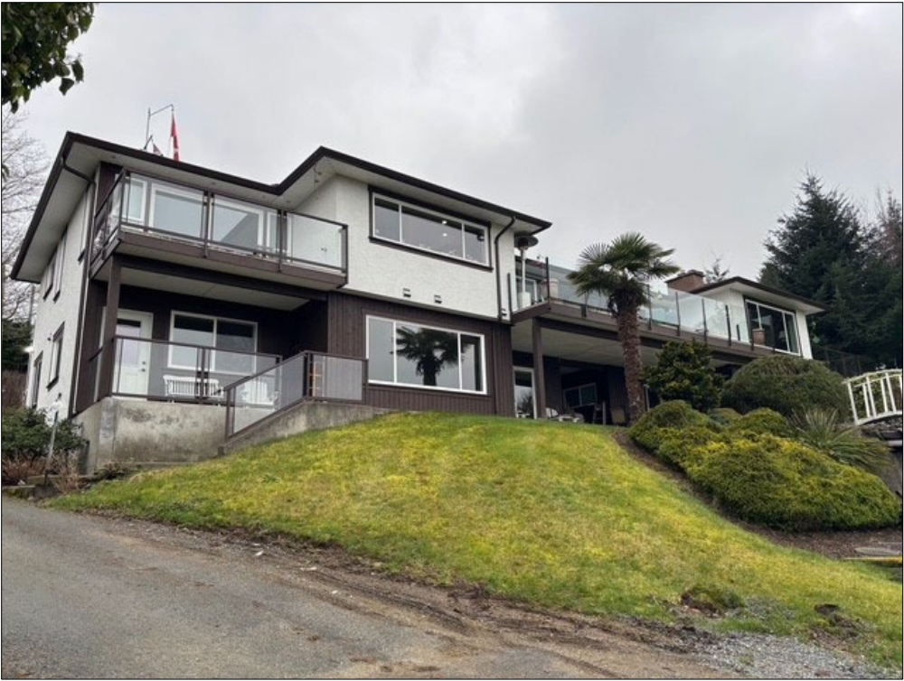
Existing principal dwelling
