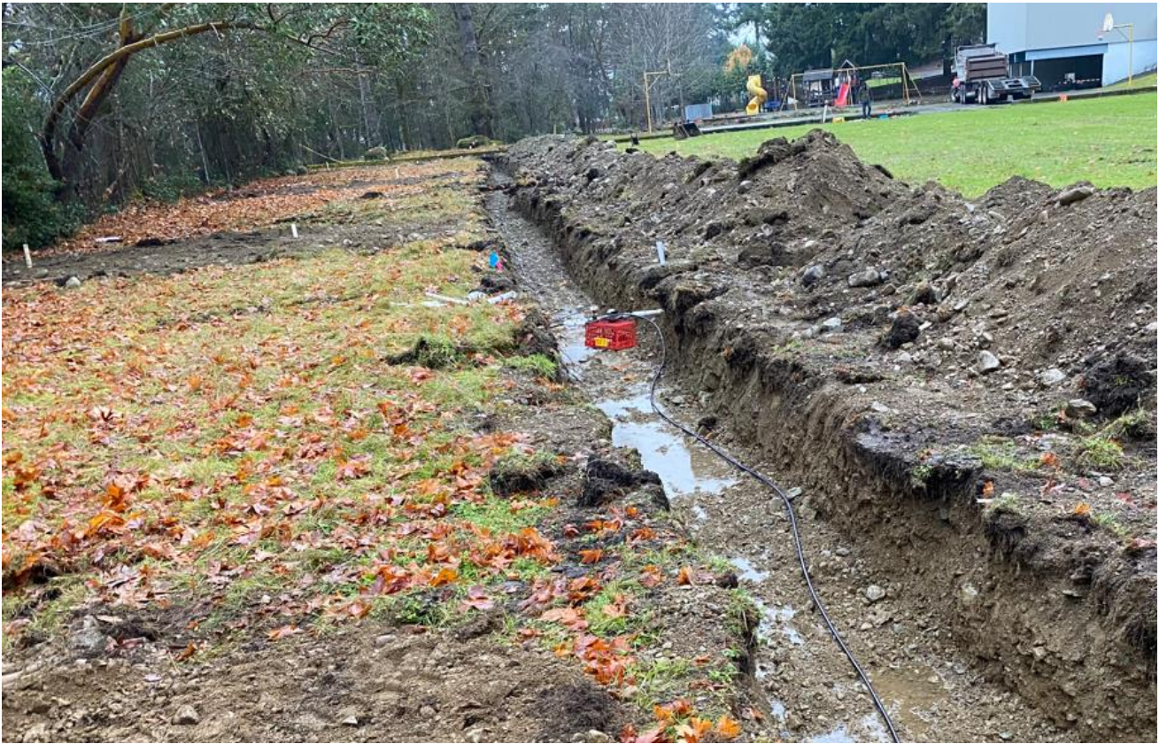
Figure 2 - Trench and Downslope Piezometers During Test Setup
