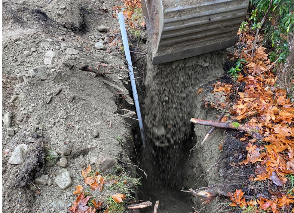
Figure 4 - Typical Piezometer Installation
