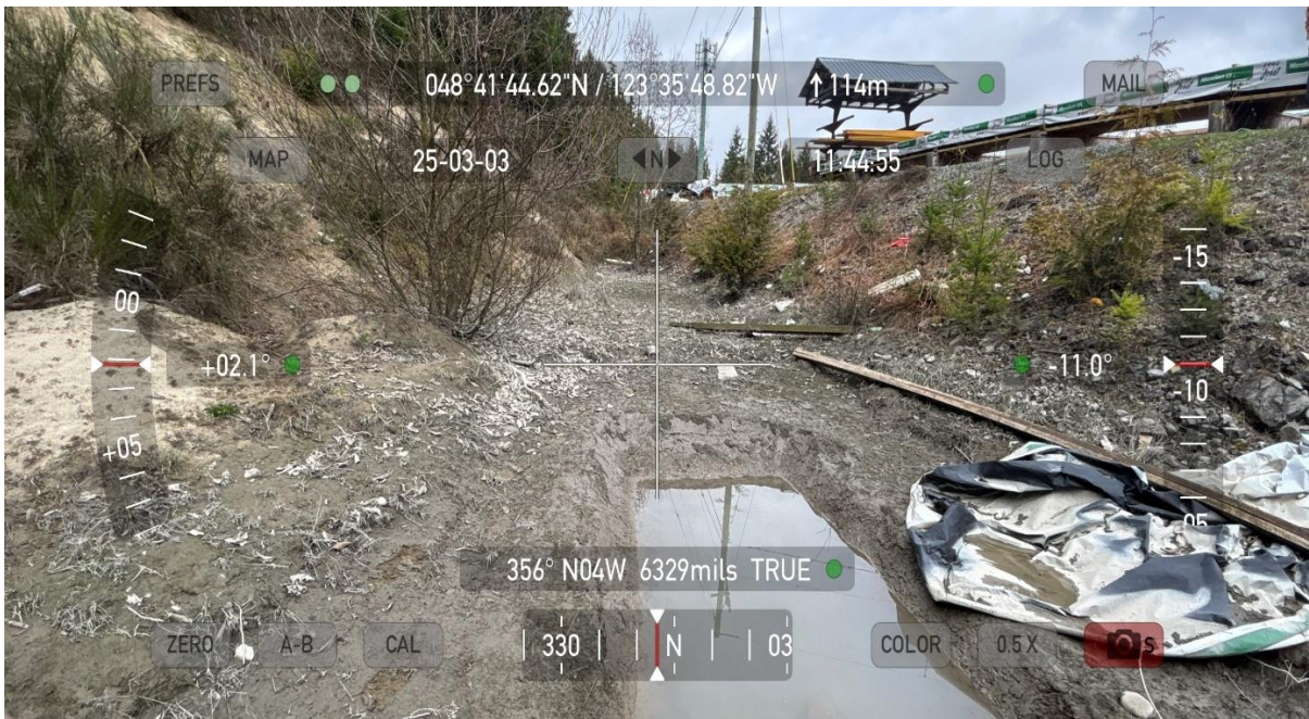
Inside infiltration ditch looking north along west property line.
