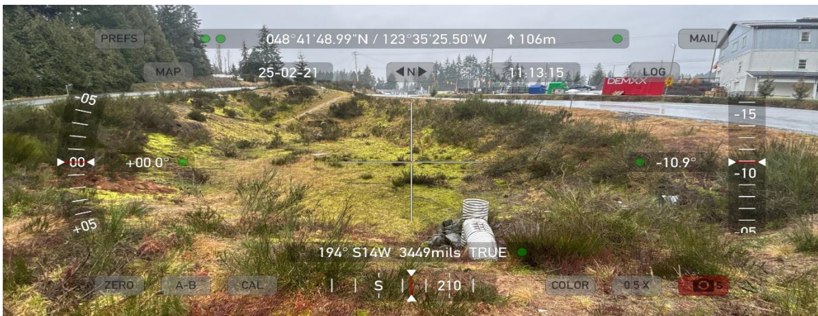
That ditch flows via culvert along with other area culverts to this retention/detention pond.
