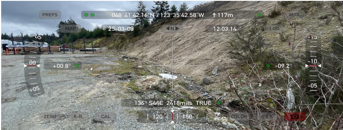
On site infiltration ditch absorbs storm water into the earth.
