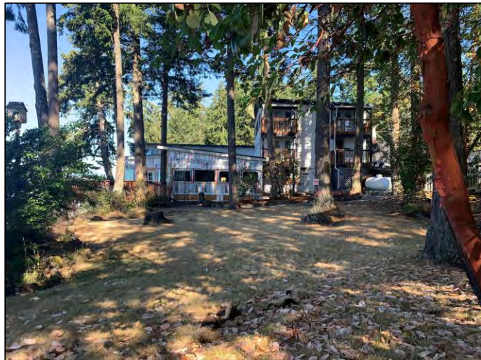
Photo 8. The side of the inn and restaurant building that is under renovation. Trees in the area to the southeast of this building are to be removed for new development.
