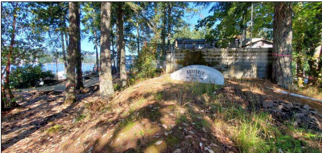
Photo 9. Trees to be removed and the concrete block fuel tank structure to be removed.
