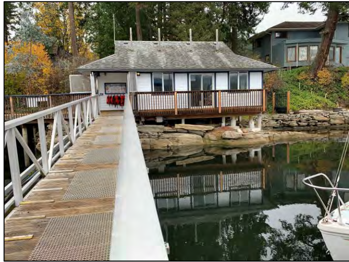
Photo 4. The marina office in the southern corner of the property is on piers above the shoreline and a gangway leads out to the existing marina docks.
