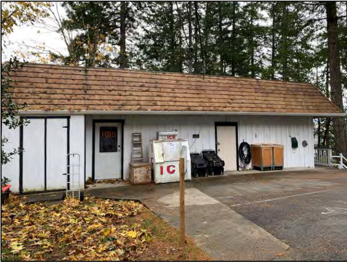
Photo 7. The existing accessory building with washrooms, laundry and shower facilities.
