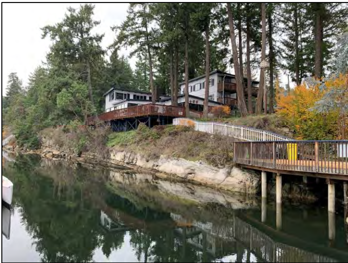
Photo 5. Another view of the shoreline with the inn and restaurant above and the pathway leading down to the decking off the marina office.
