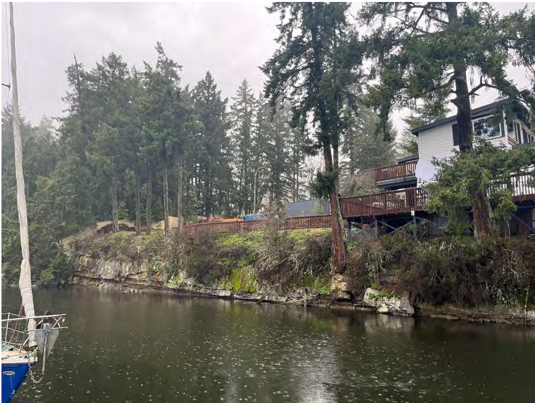
Photo 2.2.1: Foreshore area. Looking north.
