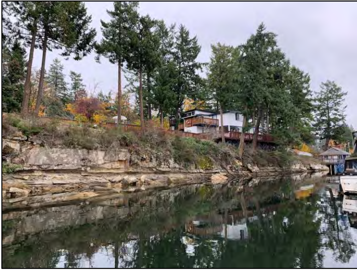
Photo 3. The property is waterfront to Ladysmith Harbour. The restaurant decking extends out towards the sandstone vertical shoreline slope.
