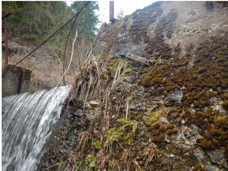
Photo 20 Downstream face as viewed from the left of the spillway.
