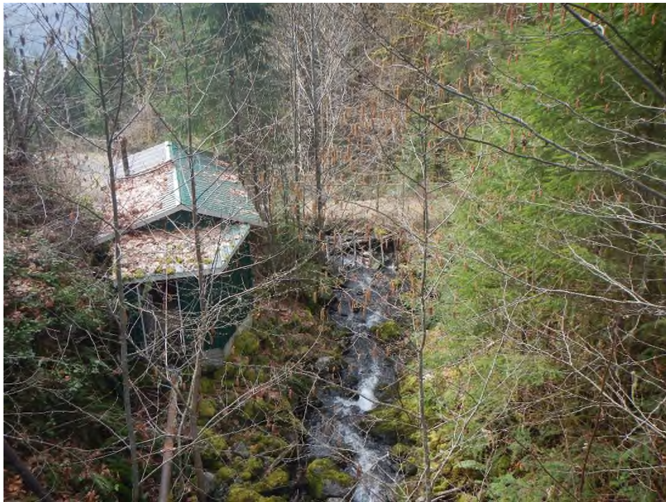
Photo 24 Outlet channel as viewed from the dam crest.
