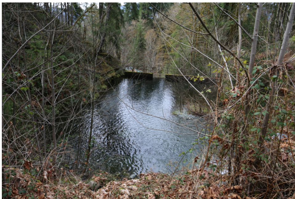
Photo 2 Reservoir as seen from the upstream side of the dam.
