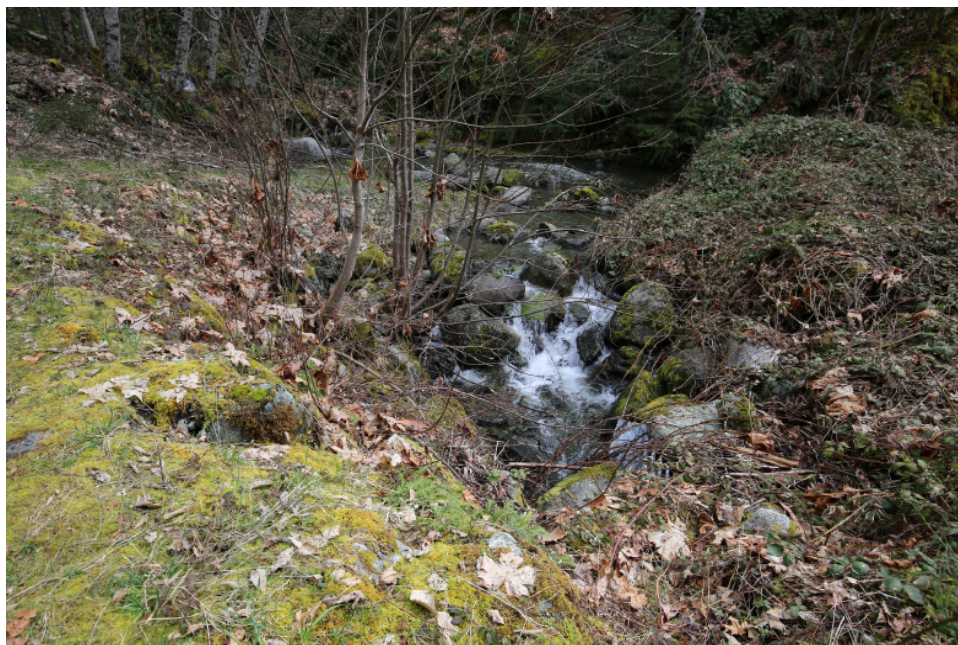
Photo 1 Upstream stilling basin and channel leading to culvert.
