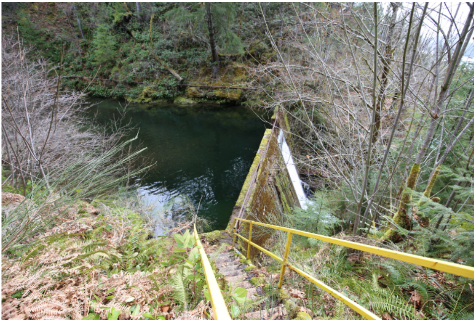
Photo 4 Right upstream access to the dam crest.
