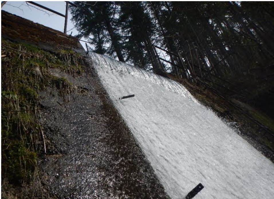
Photo 16 Water flowing over spillway as viewed from below.
