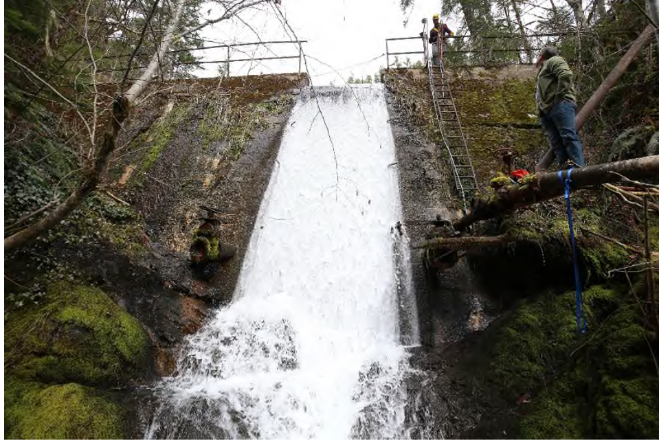
Photo 17 Downstream face of the dam as viewed from downstream.
