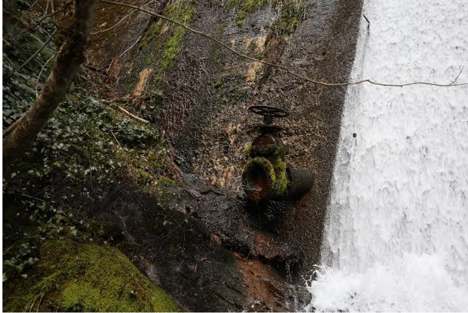
Photo 21 Low level outlet on the right side of the dam.
