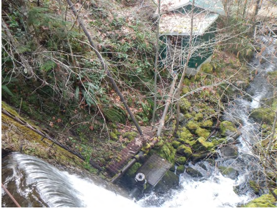
Photo 23 Low level outlet and water intake pipes viewed from dam crest.
