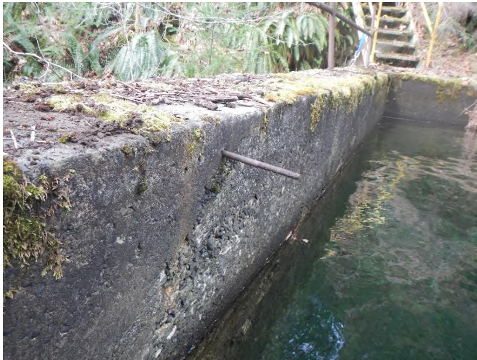
Photo 6 Upstream face of the dam above waterline.
