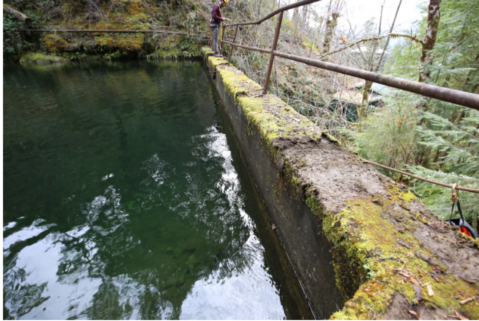
Photo 5 Dam crest as viewed from right side of the dam.
