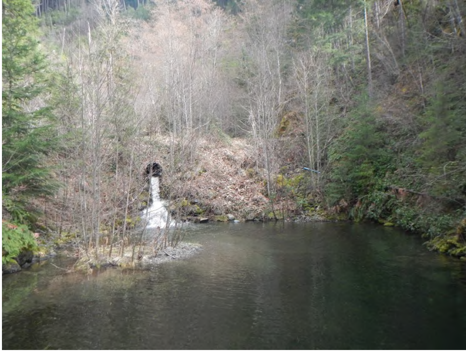
Photo 3 Culvert discharging into reservoir upstream of the dam.
