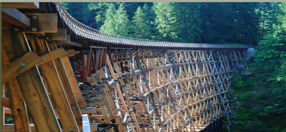
Newly rehabilitated Kinsol Trestle (2011)
