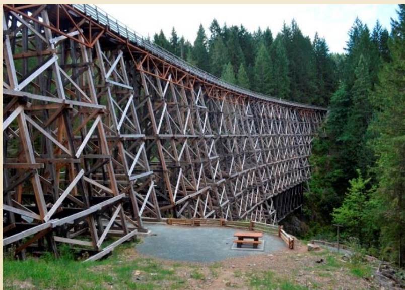
Kinsol Trestle Completed
