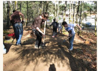
Mountain bike trail construction Cleasby Bike Park (2011)
