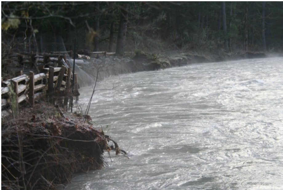
Photo 7: Example of bank erosion at Stoltz Pool Campground on 1 February 2020
