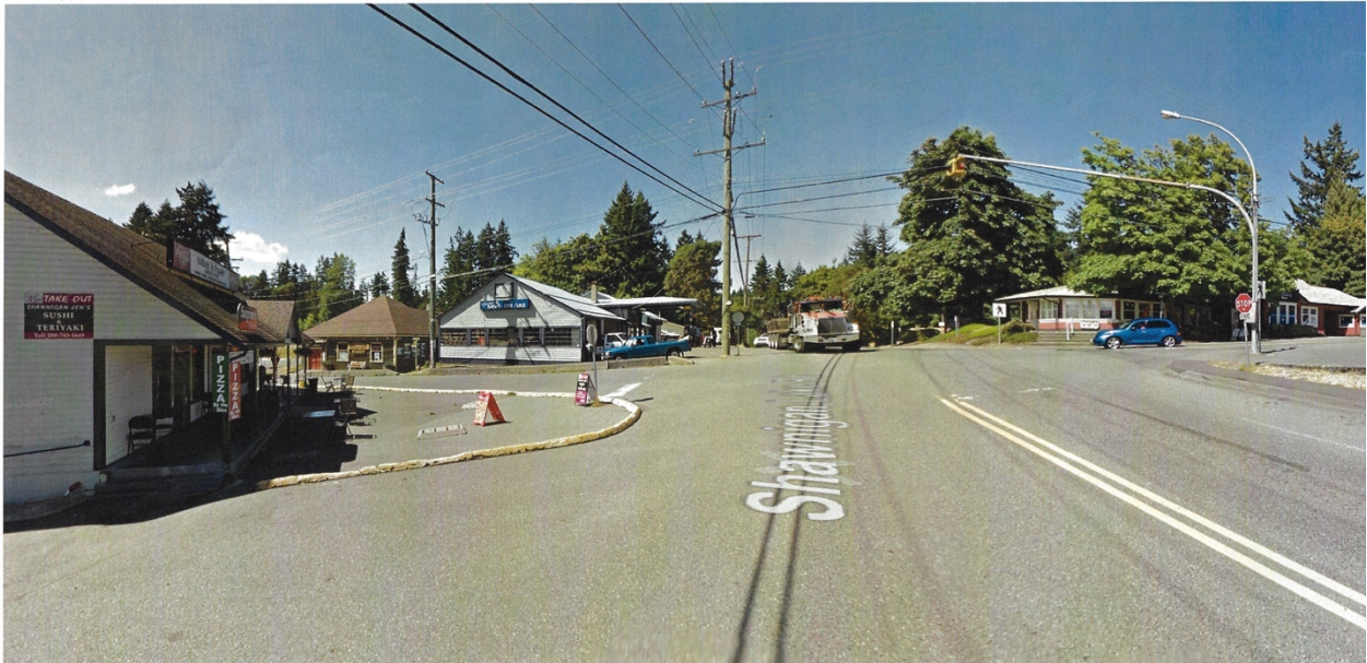
Before: Photo of existing “Four Corners” intersection in Village Core area
