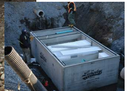
Copper Valley Oil Interceptor installation (Photo Credit: Langley Concrete)
