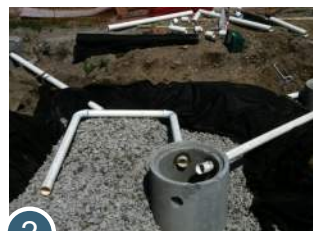
2 Rock Pit Installation, Squamish Thunderbird Subdivision
