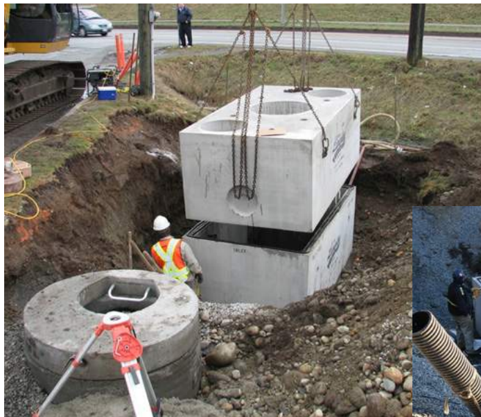
Installation of a Oil Water Separator - Coast Mountain Bus Company
