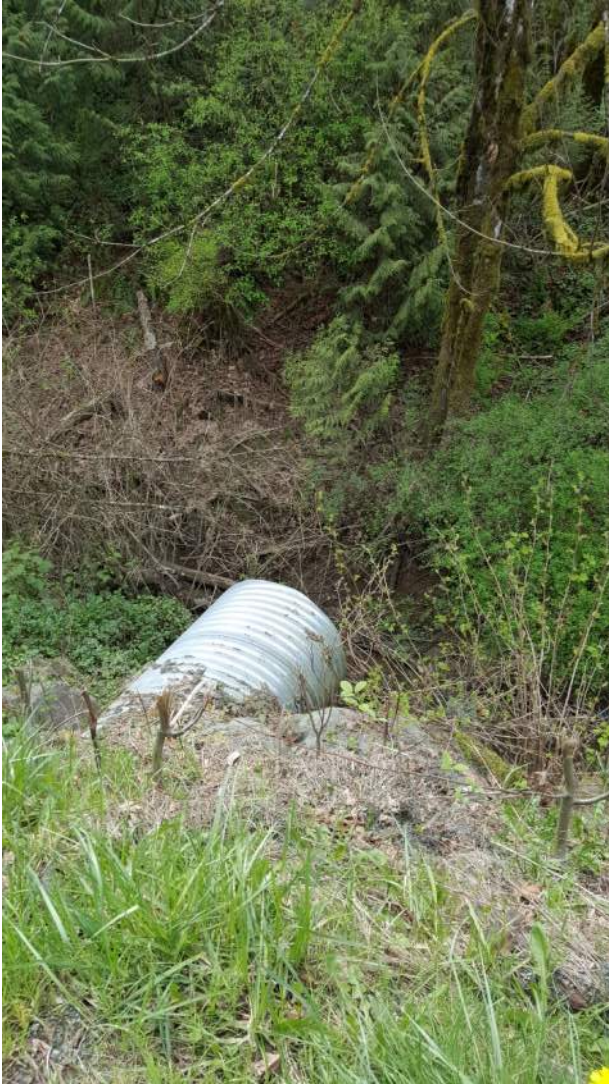
Photo 6: Miller/Koksilah Road Culvert Inlet
