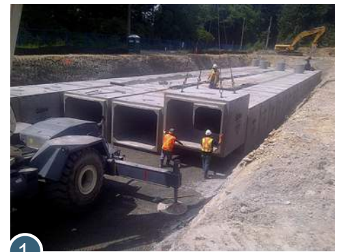
UBC Detention Tank Installation
