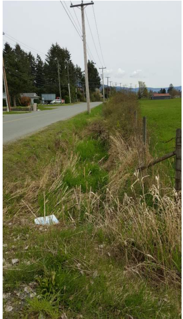
Photo 3: Glenora Road Ditch (south of the road)
