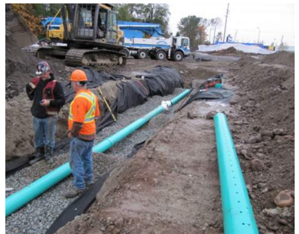
Rock Trench Installation with Perforated Pipe, MEC North Vancouver
