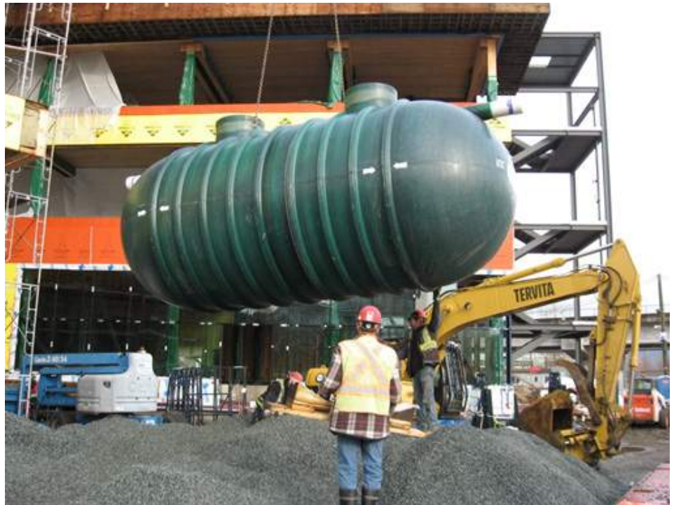
Detention Tank Installation, MEC Head Office
