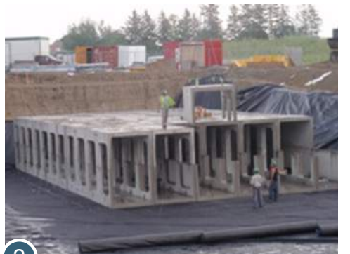
StormTrap Detention Installation (Photo credit: Sustainable Technologies Evaluation Program)
