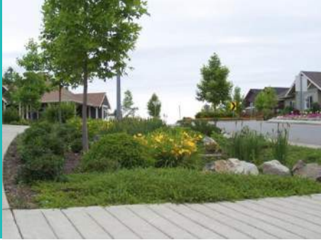
Partial infiltration swale with reservoir and subdrain
