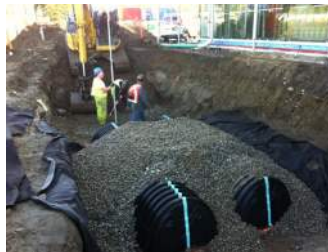
Infiltration Chamber Installation, MEC North Vancouver
