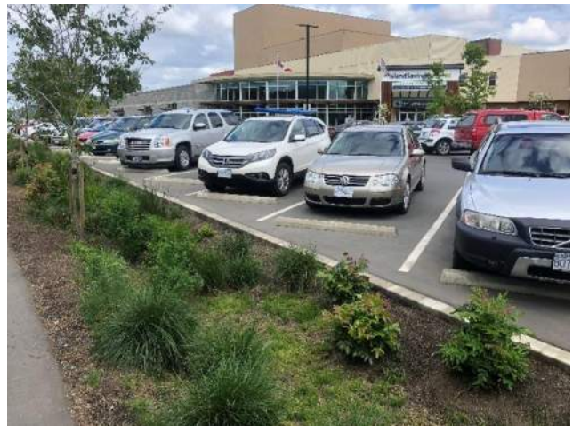
Raingarden/infiltration swale at Cowichan Recreation Center Parking Lot.
