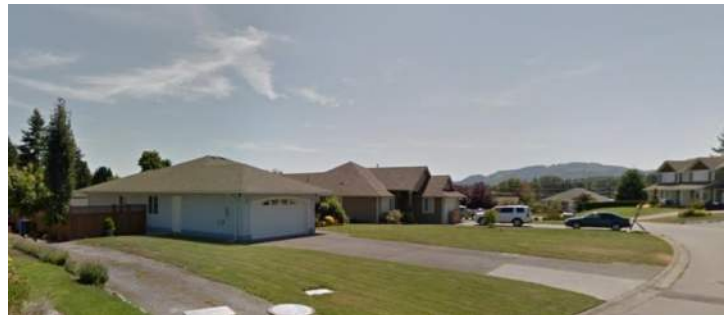
Typical existing residential area properties with curb gutter, paved driveways and lawns
