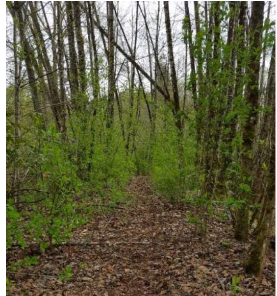
Trestle Village Dike showing mature trees and vegetation growing on dike.
