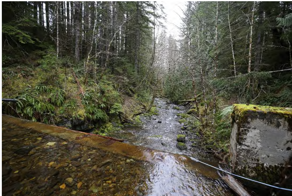
Photo 4 Dam downstream channel as viewed from upstream side.
