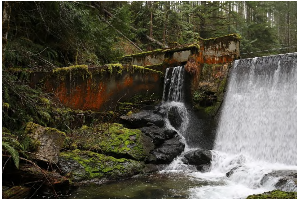
Photo 16 Right side of the structure including wingwall as viewed from downstream.
