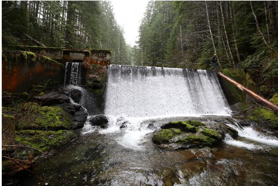
Photo 15 Downstream face as viewed from downstream.
