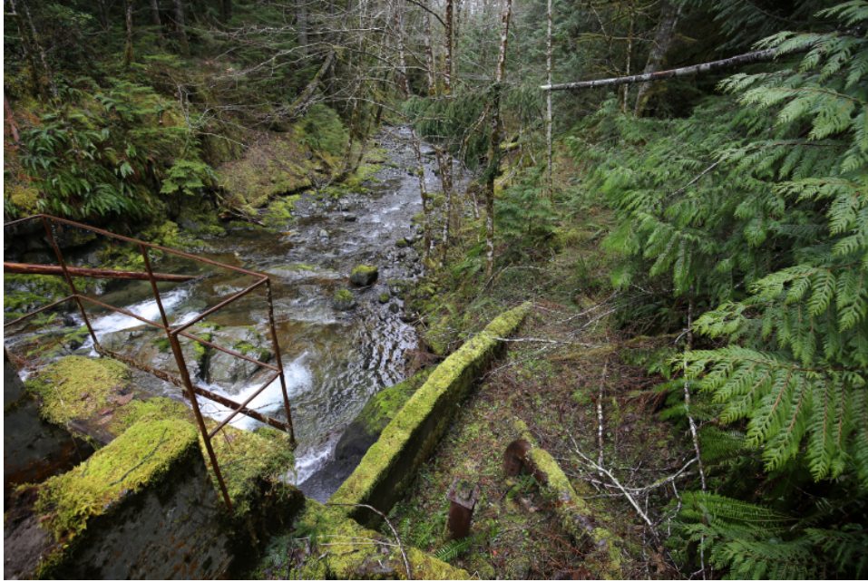
Photo 7 Downstream wingwall below spillway.
