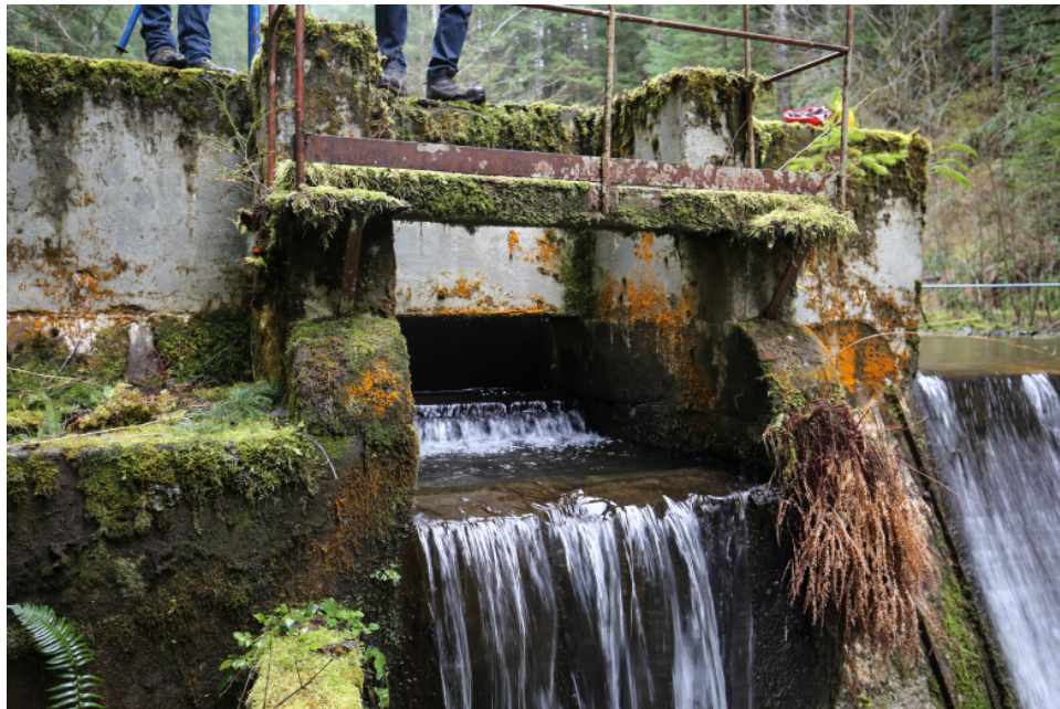
Photo 10 Small discharge channel on the right side of the dam.
