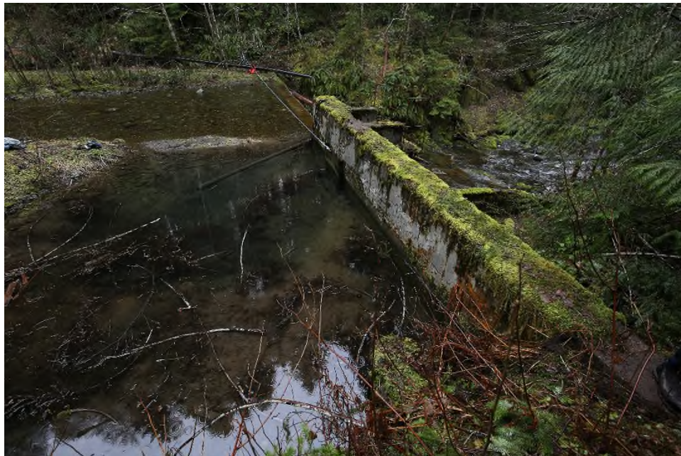
Photo 2 Dam upstream face as viewed from right abutment.
