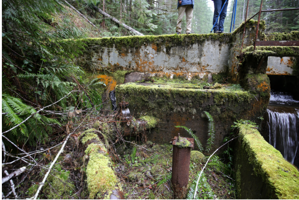
Photo 9 Low level outlet valve located on the right abutment.
