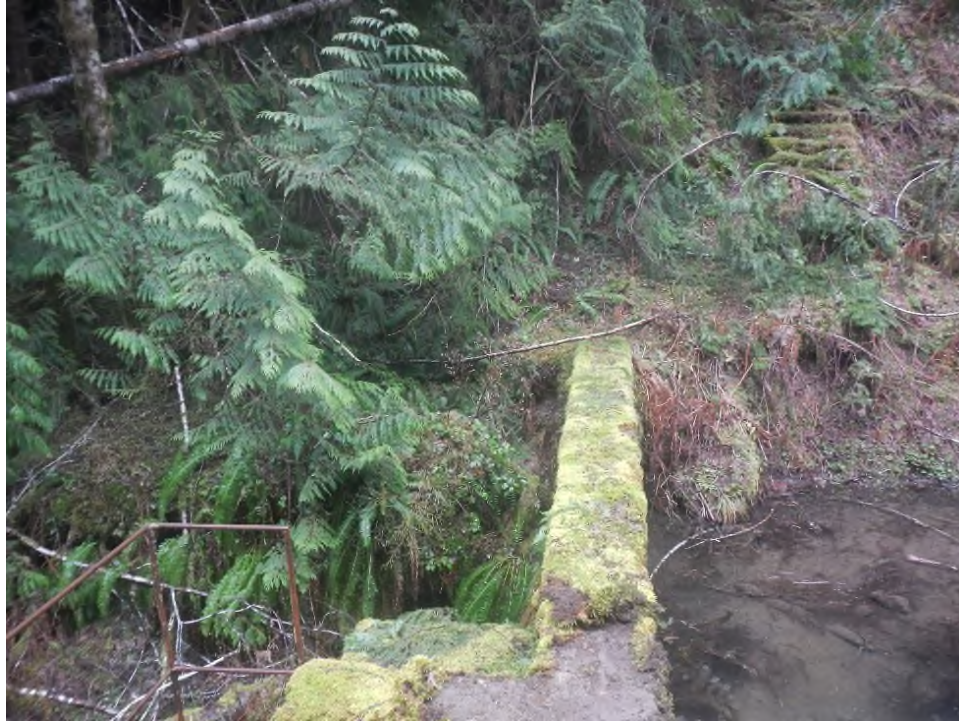
Photo 5 Right abutment and staircase used for access.
