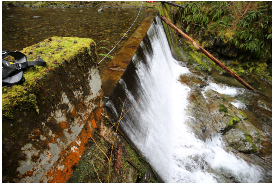
Photo 12 Main spillway as viewed from the right side of the dam.
