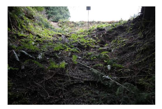
Photo 4 Sinkhole at the location of the right abutment observed in January 2018, not flowing on March 29, 2018
