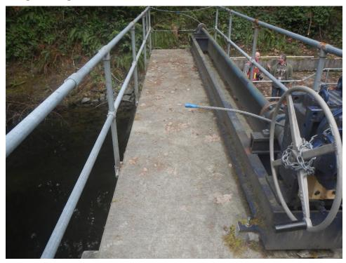
Photo 8 Walkway with cable reel above the weir.
