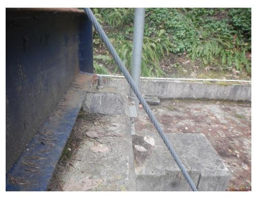
Photo 11 Crack on the grout pad underneath mechanical lift (left side).
