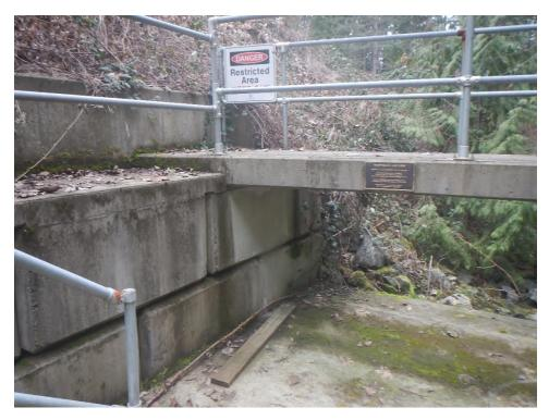
Photo 7 Retaining wall at right abutment.
