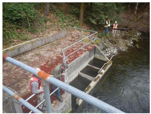
Photo 12 Mild corrosion on steel guardrail pipe connections.
