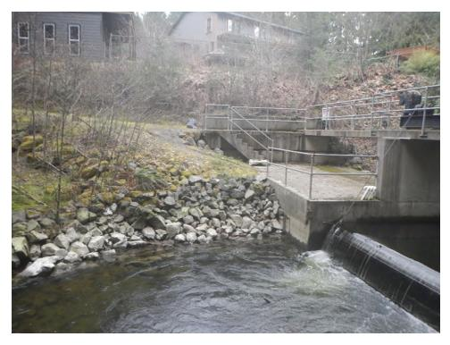
Photo 17 Riprap located on the downstream side of the weir.
