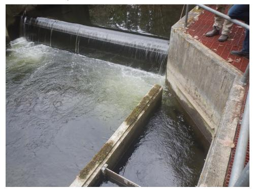
Photo 14 Moss growing on the fish bypass side wall.
