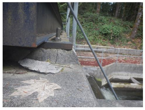
Photo 10 Crack on the grout pad underneath mechanical lift (right side).
