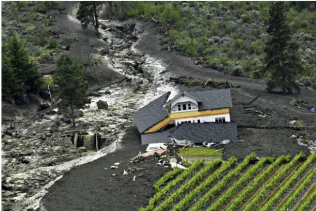
Debris from a landslide is shown from the air near Testalinden Creek, just south of Oliver, B.C. on Sunday June 13, 2010. As rescuers made their way through the debris of a landslide that struck several homes in southern British Columbia on Sunday, it began to appear that most area residents had made it out in time.
