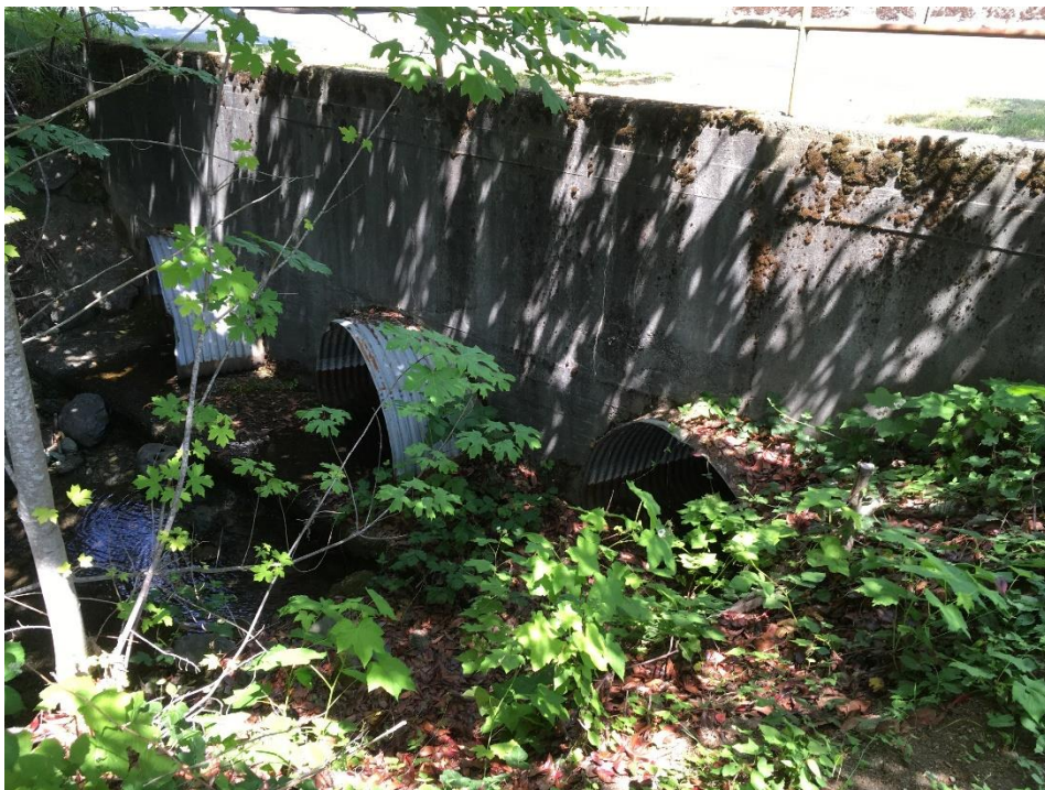
Figure 17. Culvert outlets at Youbou Creek crossing of Highway 18.
