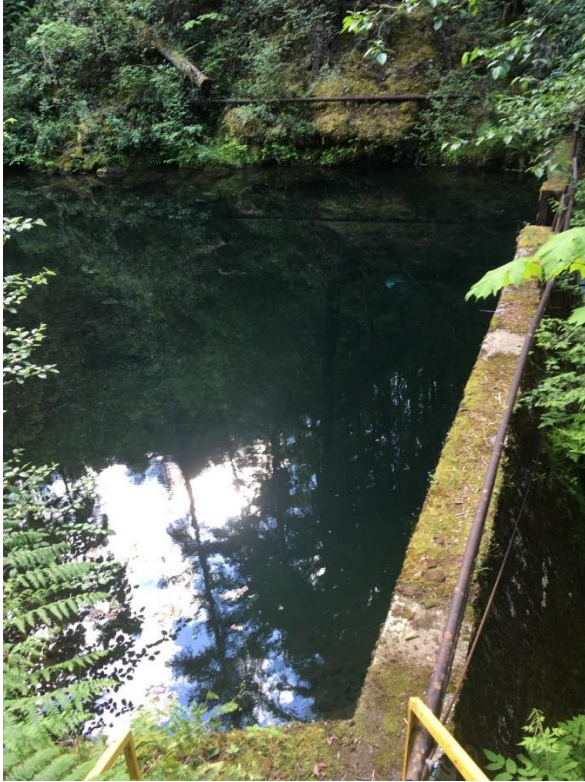
Figure 18. The dam and reservoir on Youbou Creek.
