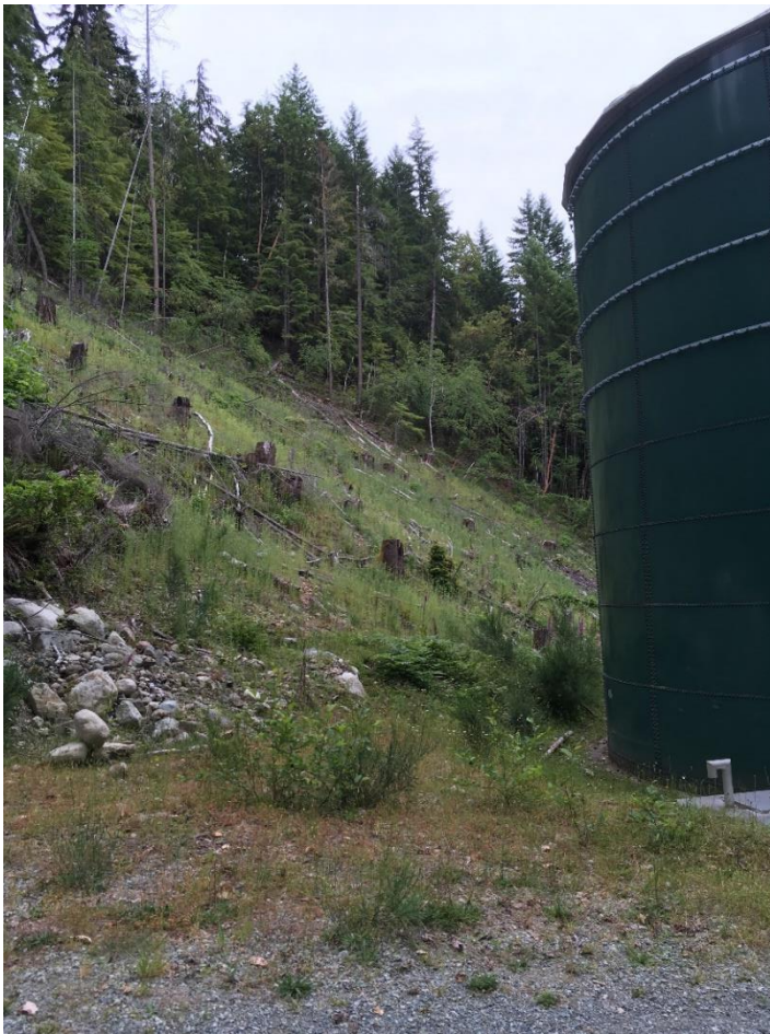
Figure 20. The water reservoir at the base of a steep, logged slope.
