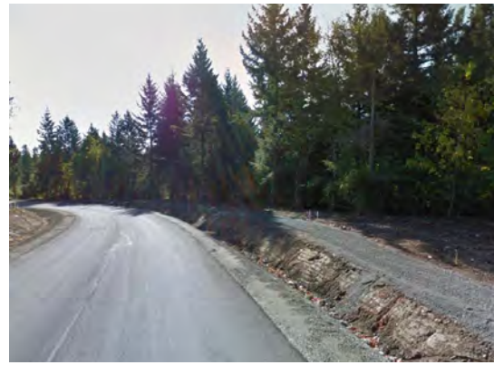
Newly Constructed Belvedere Roadside Pathway
