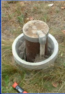
Cap with space for wiring (pitless adapter style set-up)
