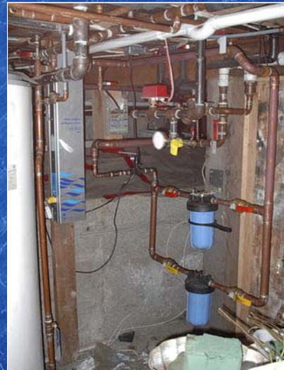
Ultraviolet Disinfection
