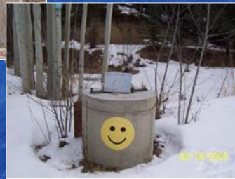
Concrete lid on dug well
