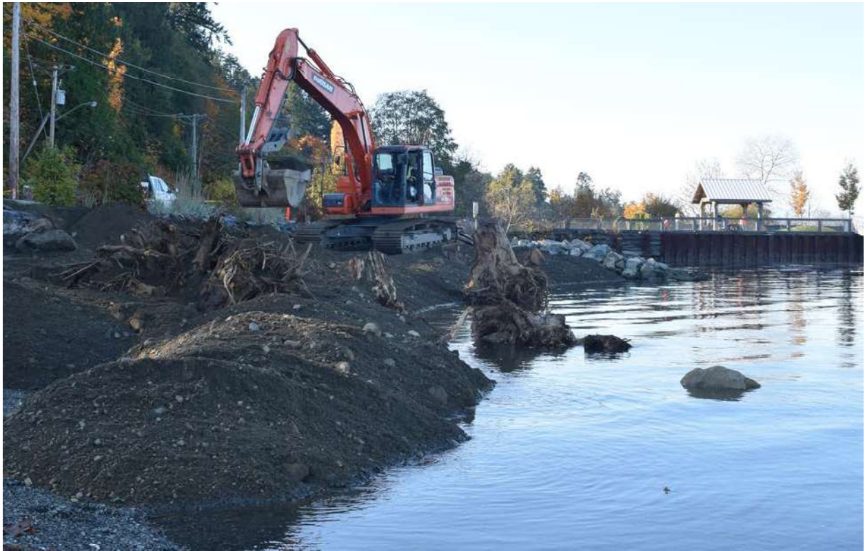
7. Contractor placing large woody debris and fish gravels at Hecate Park.
