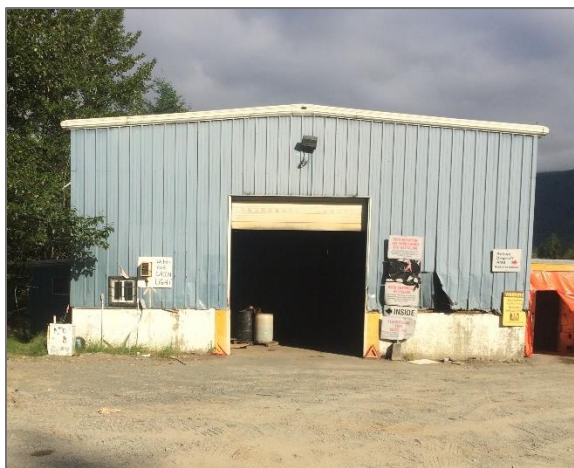
Proposed Building Prior-to Dismantling at its previous location
