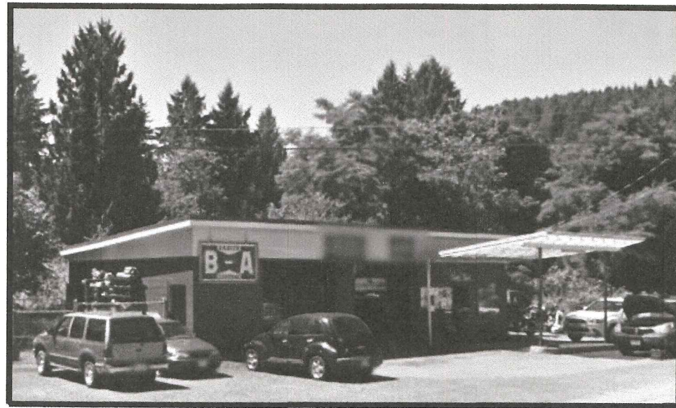
PRE-2016 RENOVATION (LOOKING SOUTHWEST)
