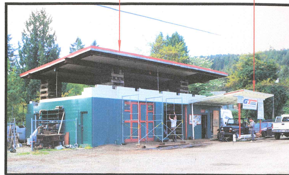
DURING 2016 RENOVATION (LOOKING SOUTHWEST)
