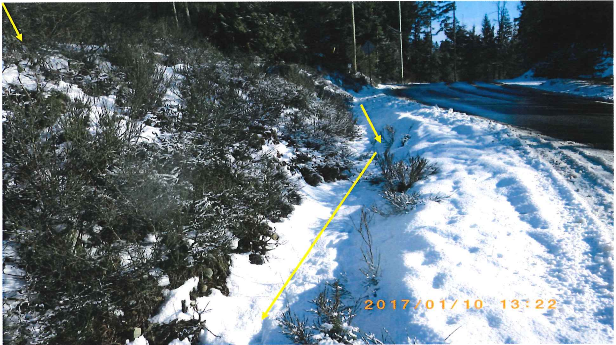
Figure 13. Looking east along the drainage ditch adjacent to Ark Road. Shawnigan lake Road lies at the end of Ark Road. Note the broom covering the side slope. The yellow arrow shows the direction of runoff flows. Photo taken January 10, 2017.
