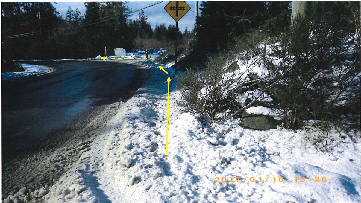
Figure 15. Looking west along Shawnigan lake Road. The drainage ditch and direction of flow is shown by the solid yellow arrow. The dashed yellow arrow is the location of the culvert under Ark Road. Photo taken January 10, 2017.
