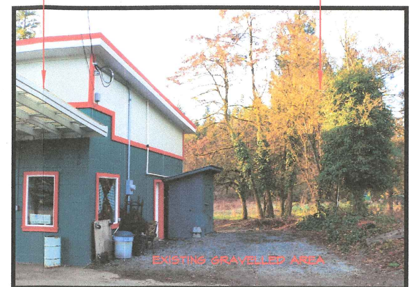
COMPLETED 2016 RENOVATION (LOOKING SOUTH, SHOWING PROPOSED WEST BAY AREA)
