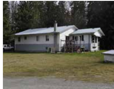
Rear of Caretakers Residence
