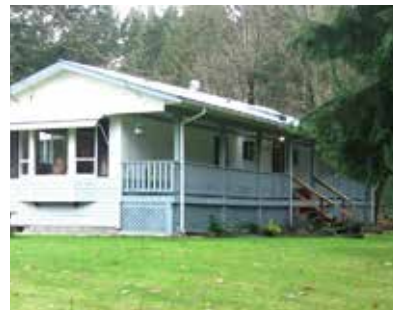
Front of Caretakers Residence
