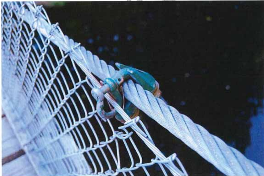
Figure 19: Makeshift Cable Connectors
