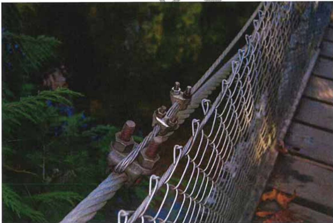
Figure 13: Additional Hand Rail Cable Connection at Mid Span
