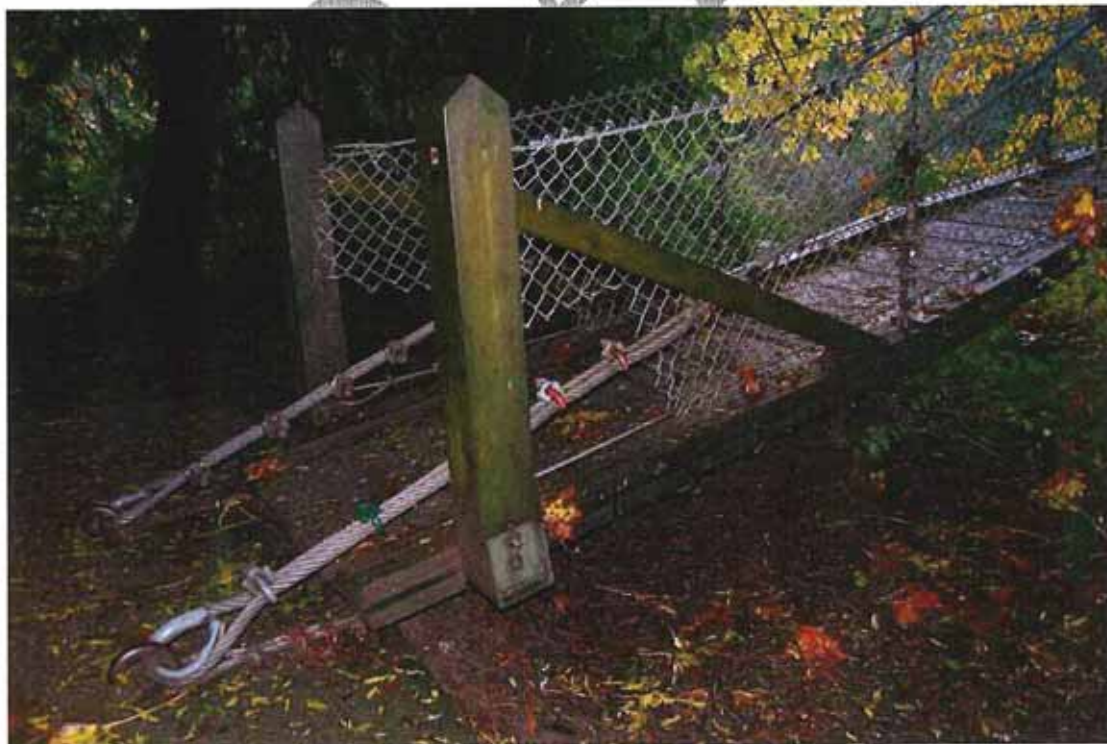
Figure 4: Cable Terminations at East Anchor
