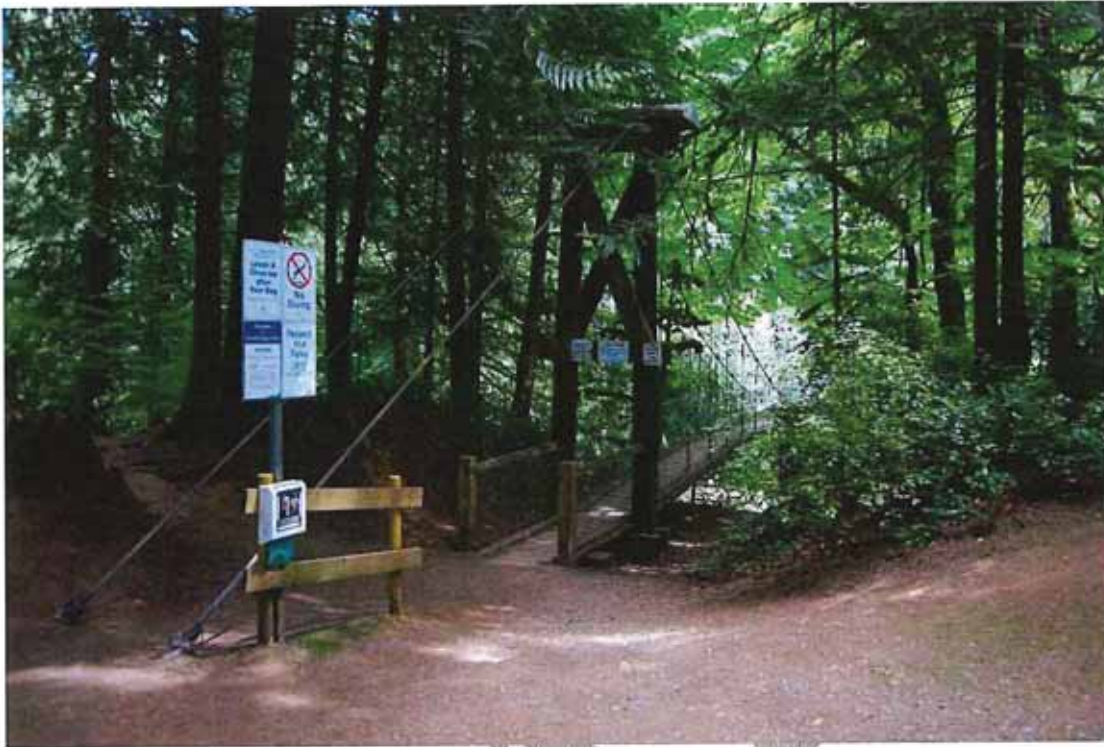
Figure 1: West Bridge Approach
