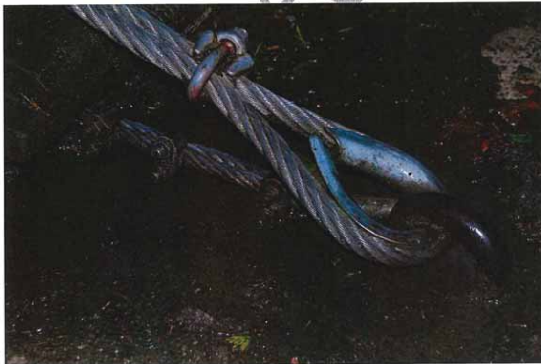
Figure 16: : Improperly Clipped Turn-Back Eye with Thimble
