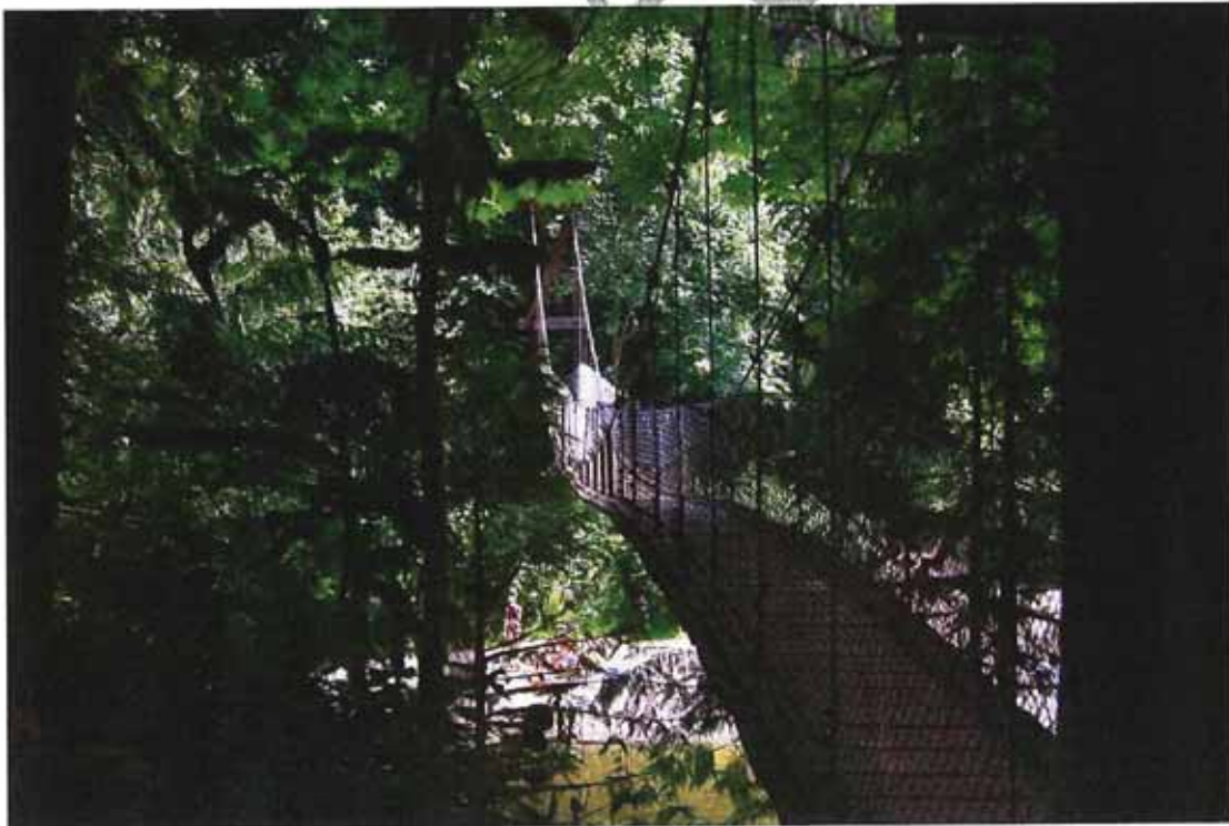
Figure 2: View of Bridge from West Approach
