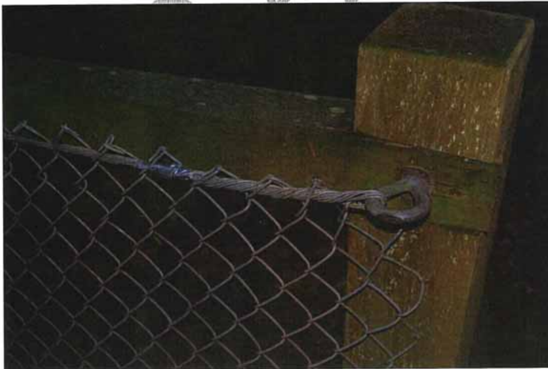
Figure 12: Spliced End Connection At Hand Rail Cable
