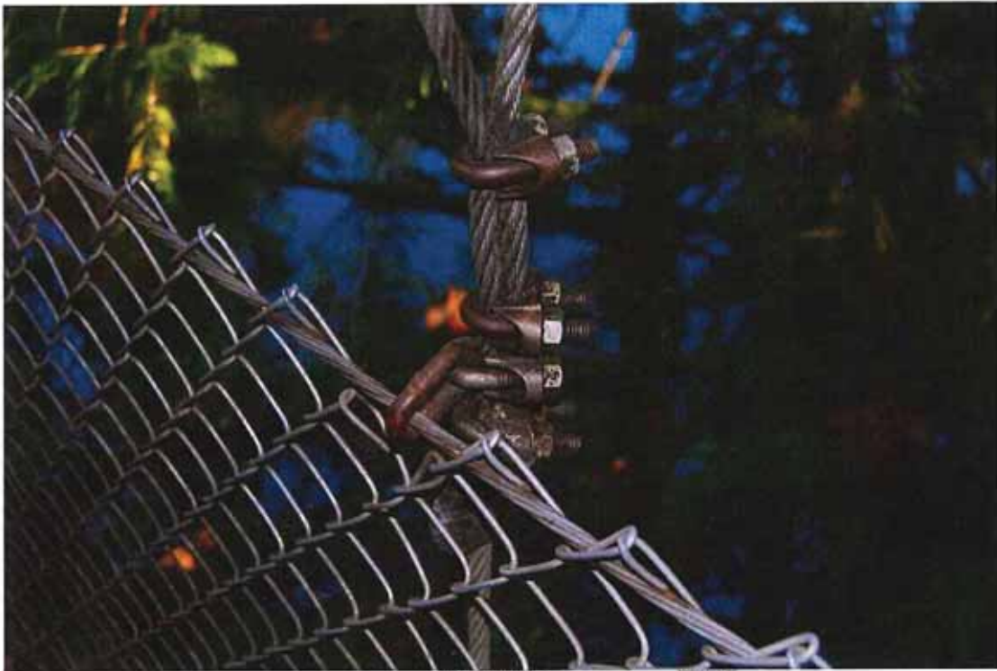
Figure 13: Typical Hand Rail Cable to Hanger Connection
