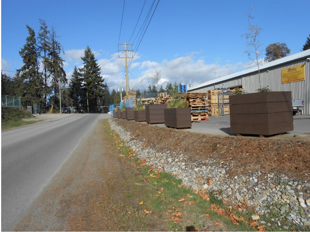
Renovation to Fisher Road building complete, new tenant, and planters installed for landscaping. Planters contrary to DP Permit
