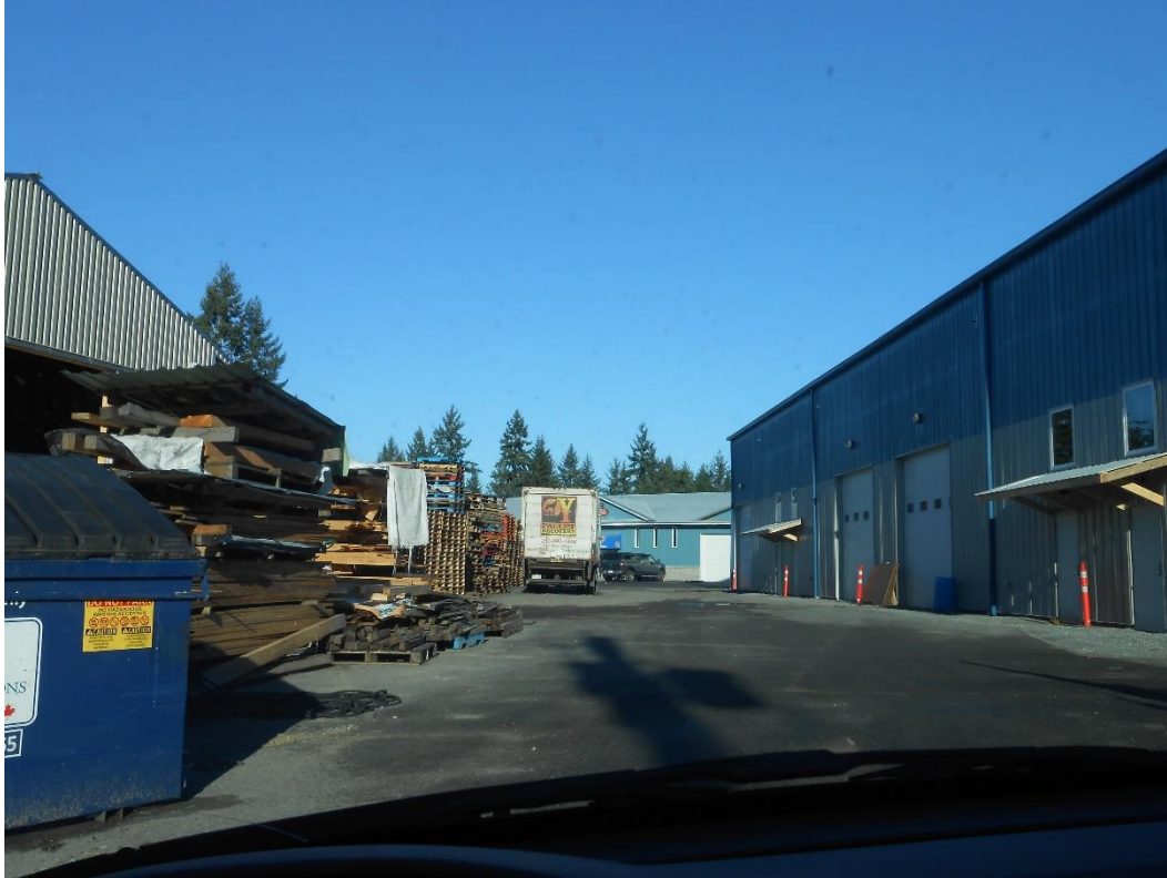
Ball Road warehouse canopies installed, no cedar panelling
