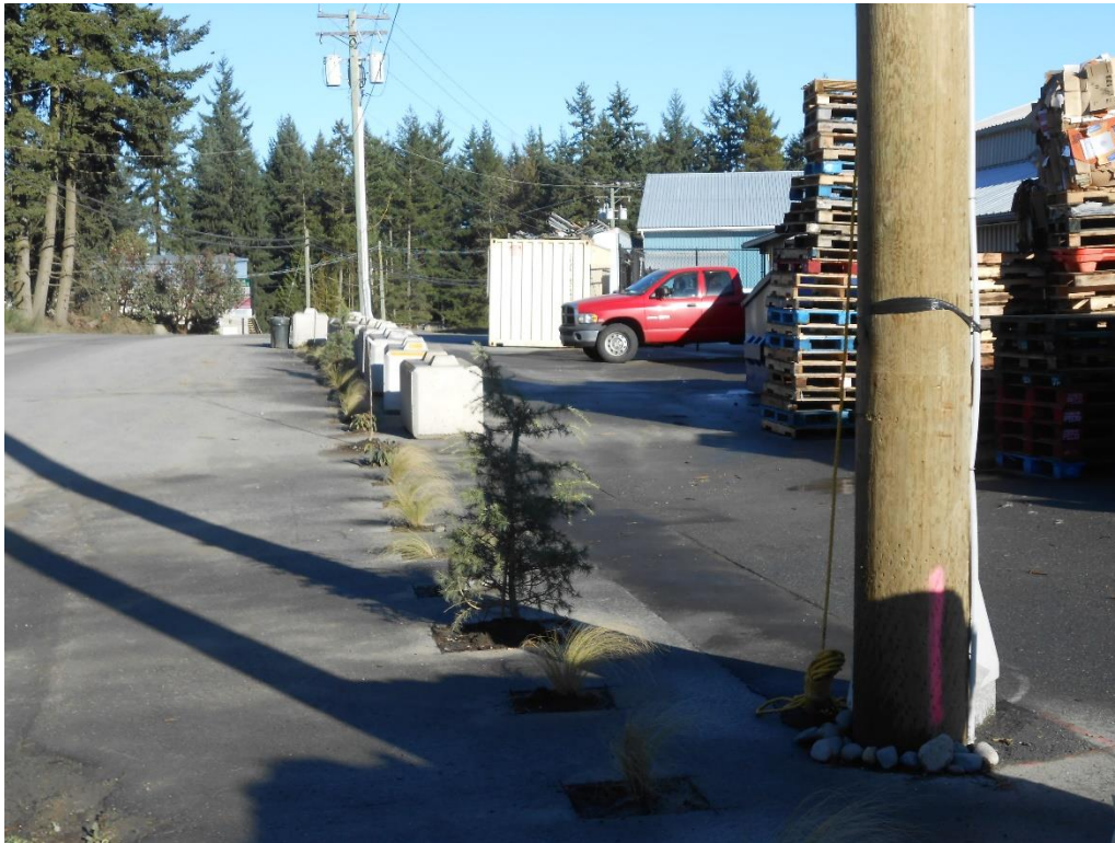
Fisher Road Frontage Landscaping Installed (December 2017)
