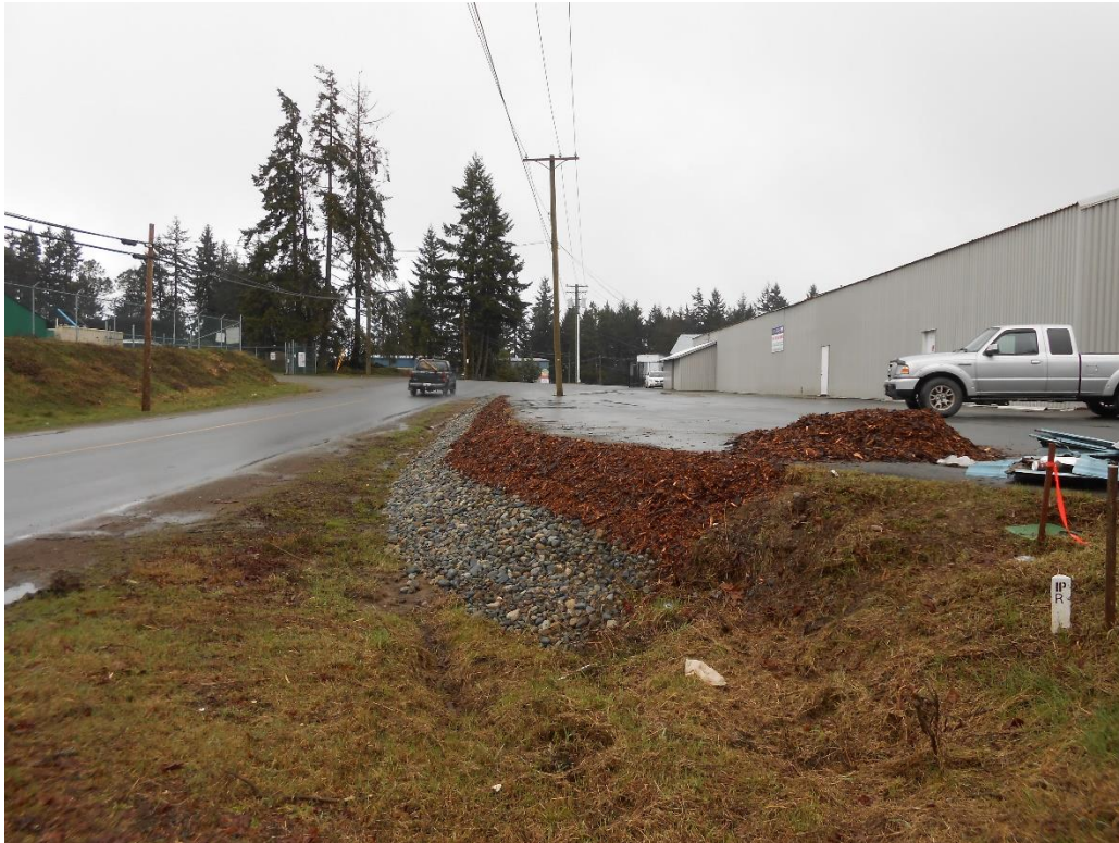
Fisher Road frontage pre- renovation (February 2016)
