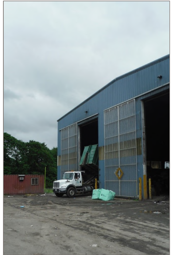
Photo 1: CVRD Roll-off truck dumping in the Transfer Building.
