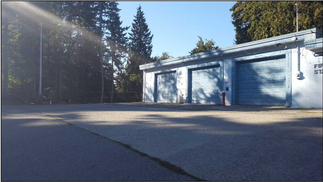
Photo 1. Showing the North Oyster Fire Station fronting Yellow Point Road and the forested area to the west where the new building construction is planned.
