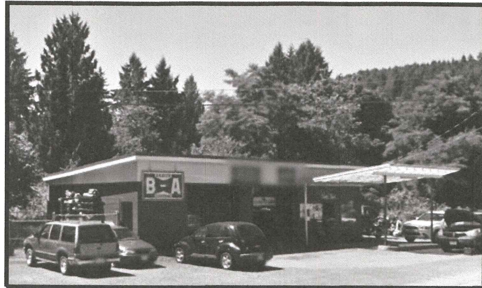
PRE-2016 RENOVATION (LOOKING SOUTHWEST)
