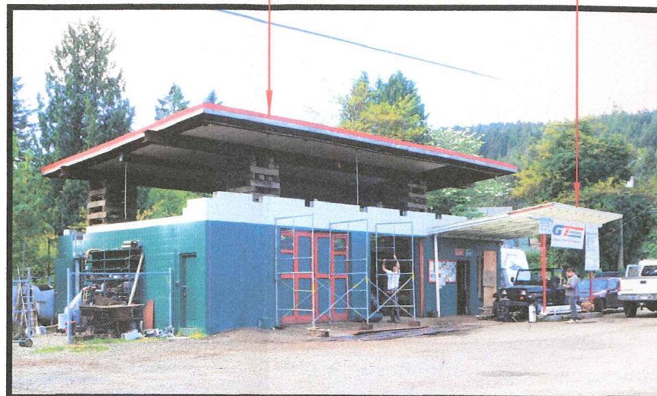
DURING 2016 RENOVATION (LOOKING SOUTHWEST)
