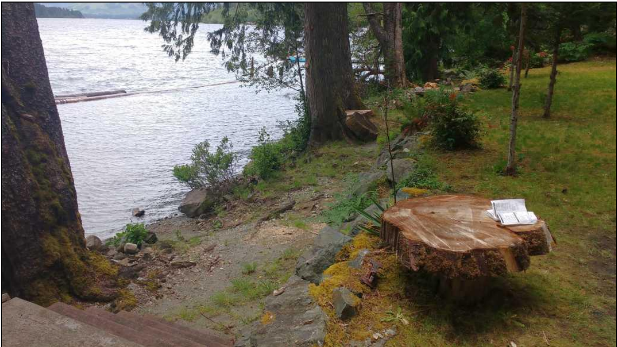
Photo 17 – Looking west along the first riprap retaining wall along the lakeshore.
