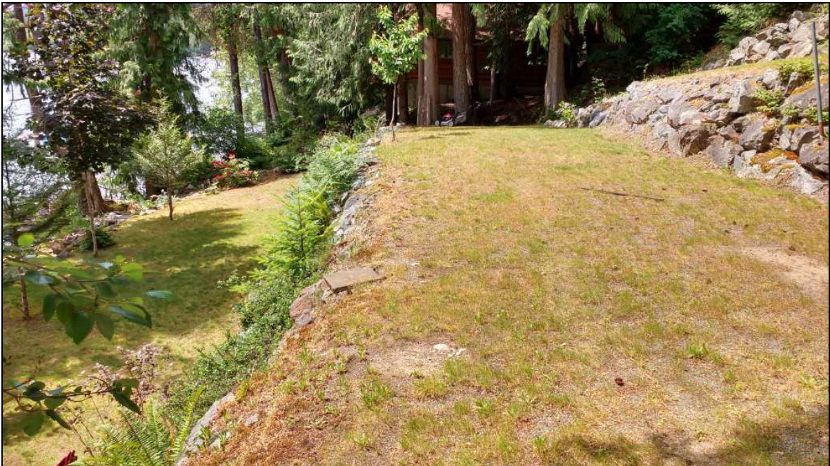
Photo 13 – Looking west along the top of the second riprap retaining wall up from the lake.
