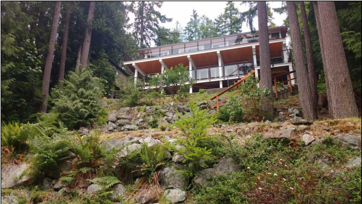
Photo 10 – Looking upslope towards the house from the base of the third riprap retaining wall up from the water's edge.
