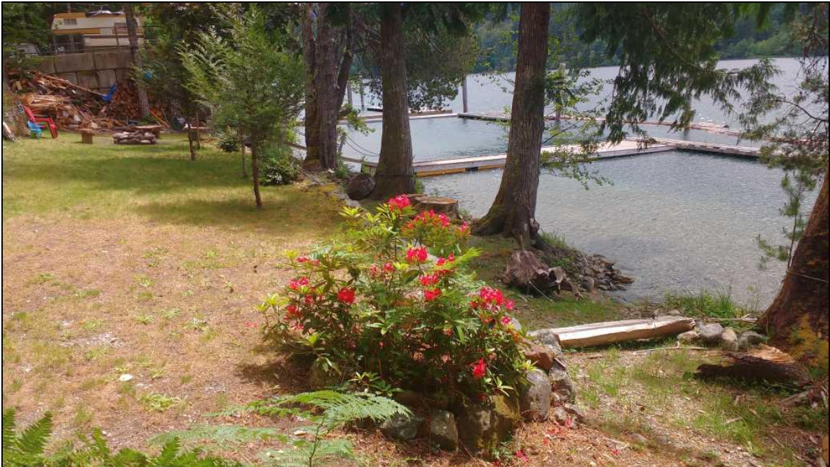
Photo 18 – Looking east along the first terrace and second riprap retaining wall up from the lake.
