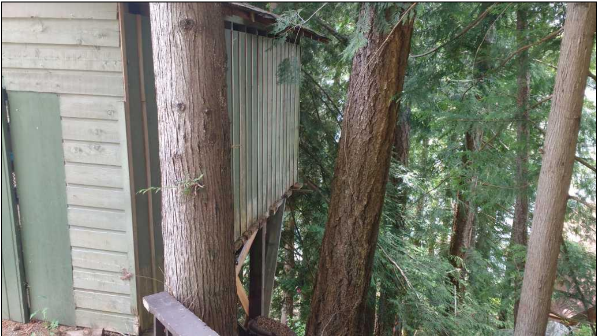
Photo 2 – West side of the existing garage, looking downslope from the front.
