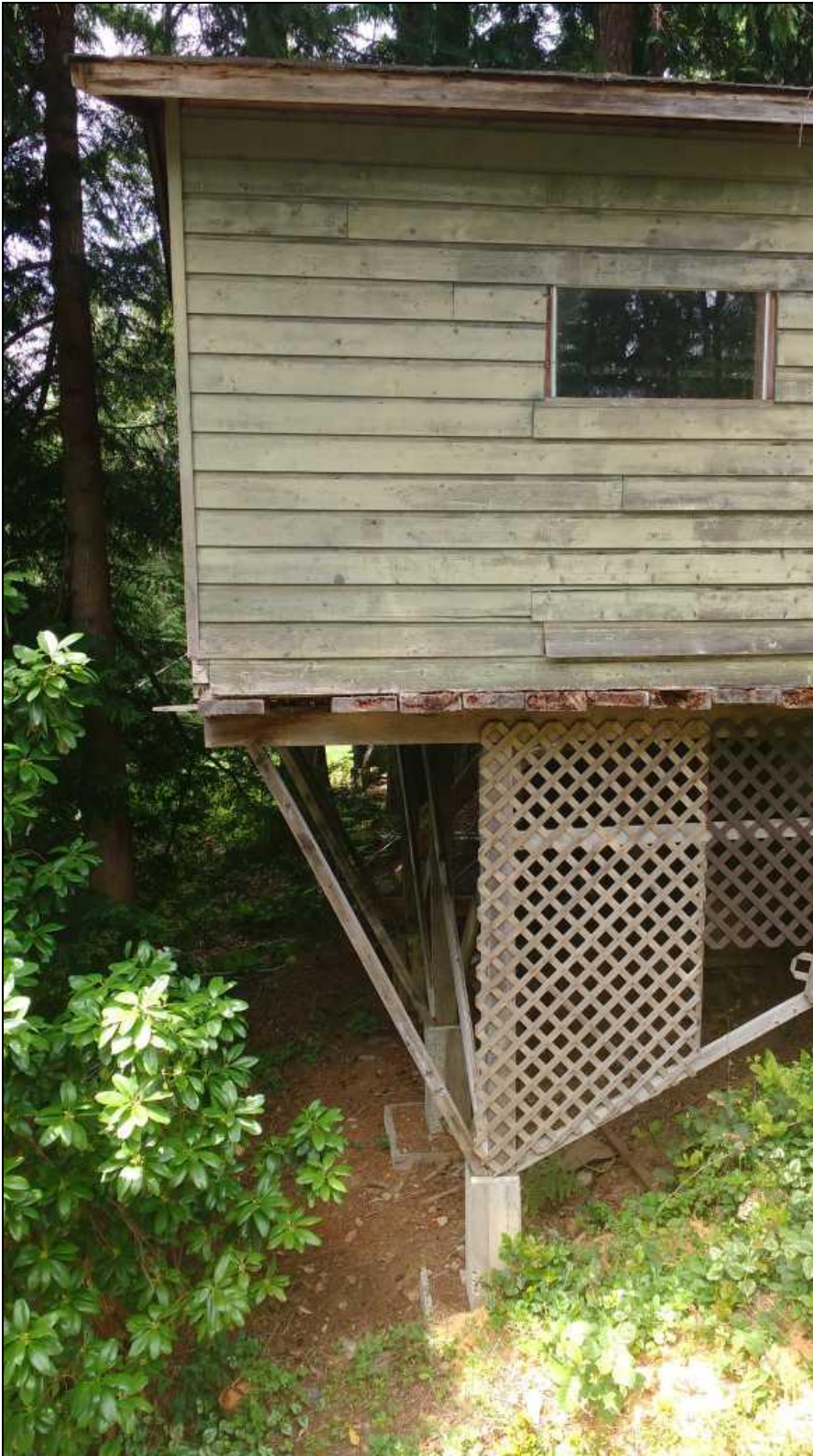
Photo 3 – East side of the existing garage.
