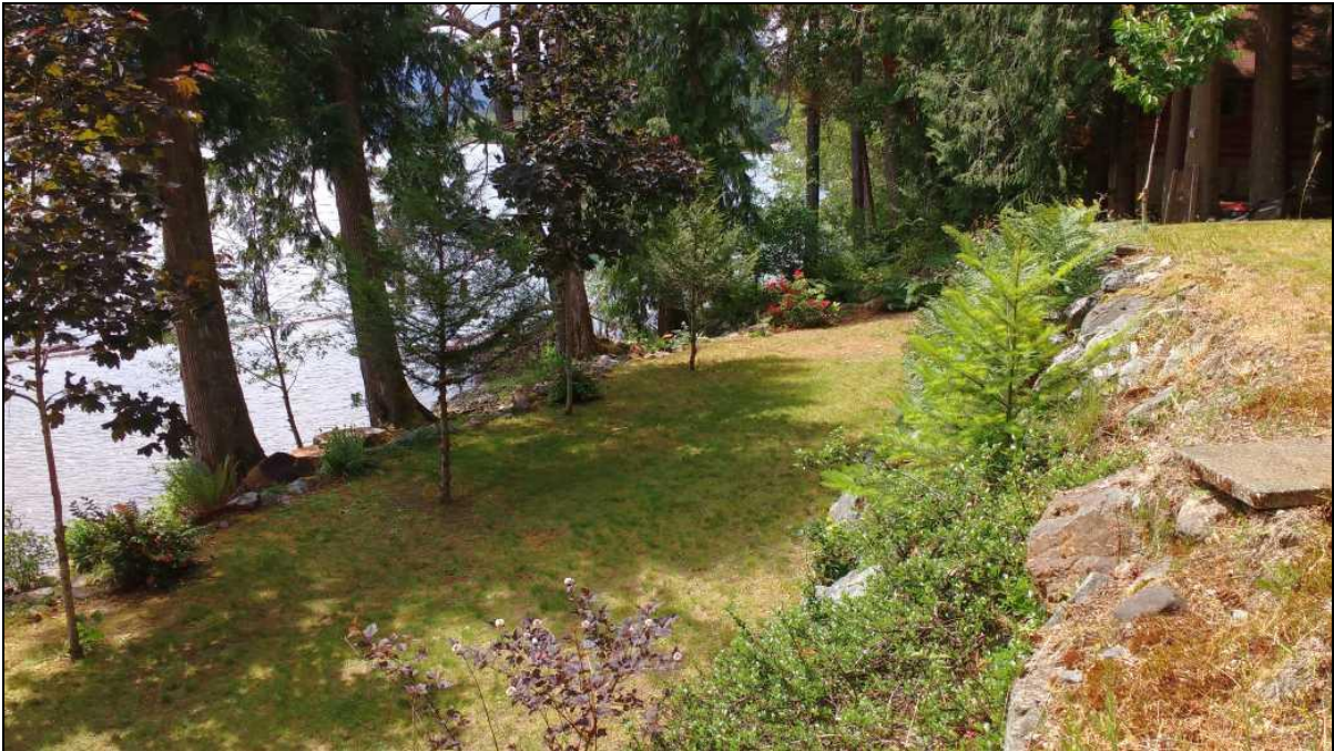
Photo 15 – Looking west along the first terrace and second riprap retaining wall up from the lake.
