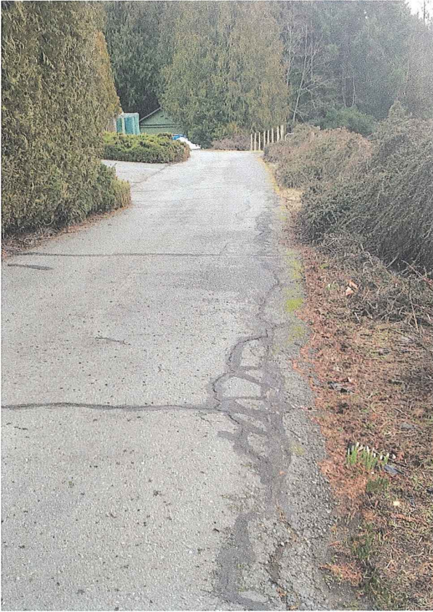
FRONT PAVED DRIVEWAY FACING EAST
