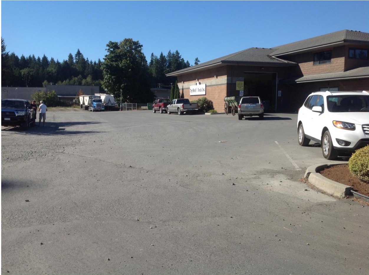
Figure 3: Looking south-west from the northern boundary at existing retail activities.
