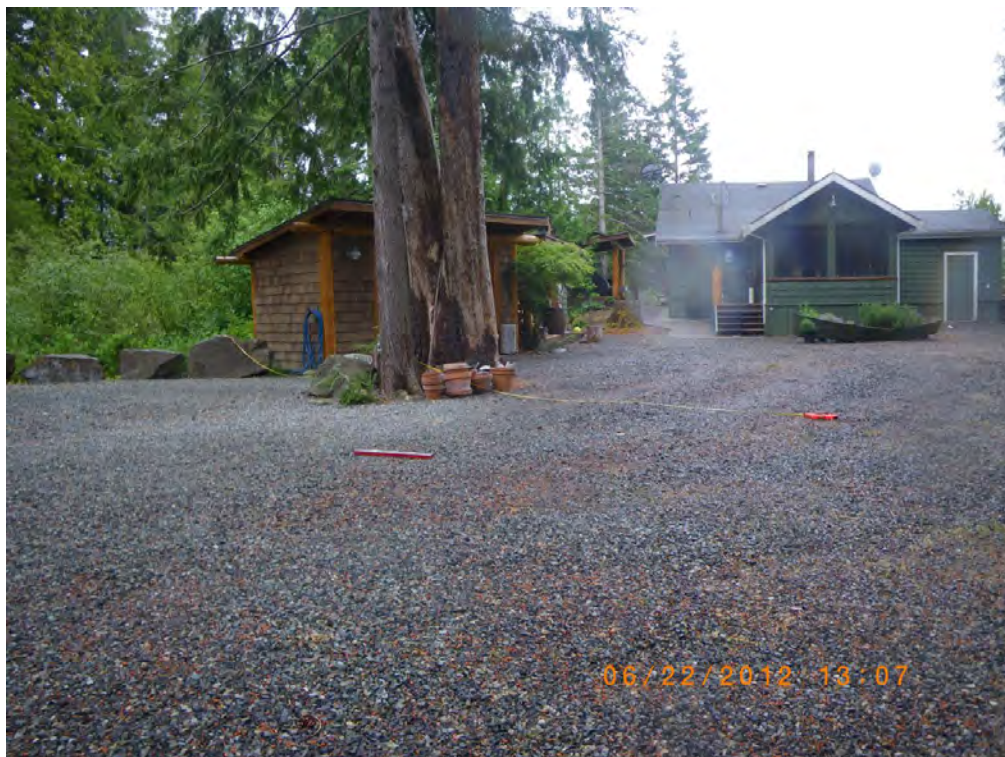
Figure 9. Photograph of the north side of the existing house and the location of the proposed building extension in the gravel parking area. An existing shed and BBQ area are visible to the left of the house (Photograph taken June 22, 2012).
