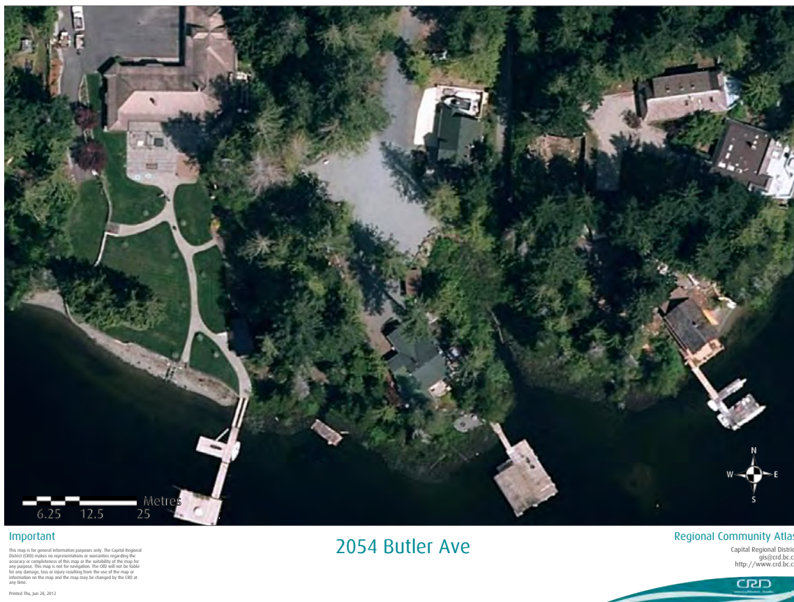
Figure 3. Aerial view of the dense shoreline riparian vegetation surrounding the rocky knoll promontory. Note the extensive gravel driveway and parking area immediately north of the existing house. Contrast the dense native riparian-wetland vegetation and conifer cover on the property with that of the development immediately adjacent to the west.
