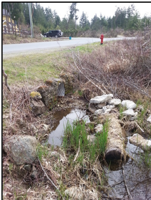
A representative photo of the outlet of the CMP that directs stormwater runoff onto the subject property.
