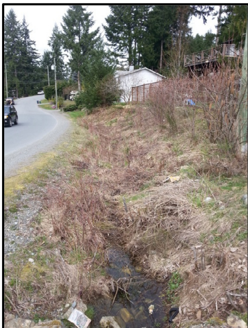
Looking north along the roadside ditch that runs parallel to Meadowview Road. Water is directed onto the subject property, from the roadside ditch via a CMP.
