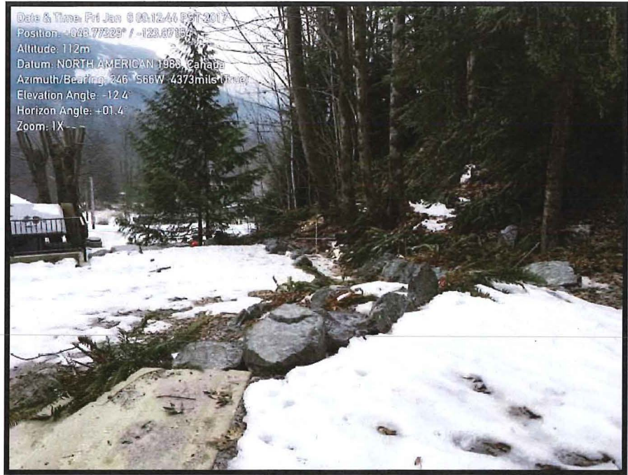
Figure 1: View towards the retaining wall from the pond.
