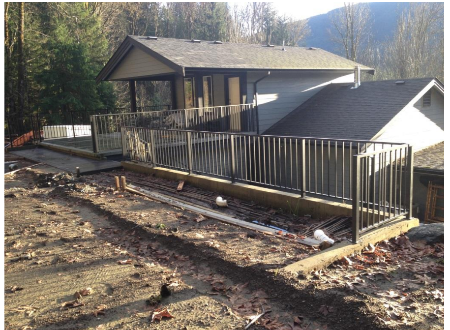
Shop & Garage looking south
