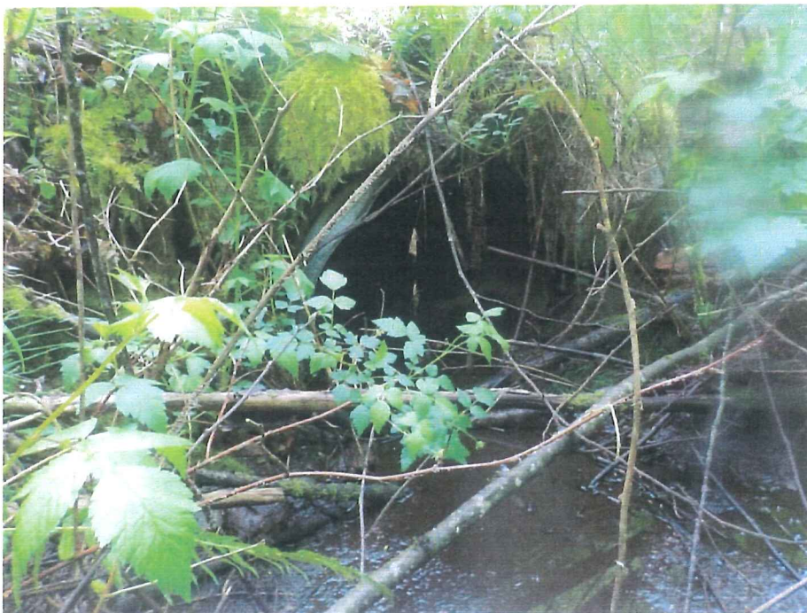
Outlet of the culvert carrying water from the wetland pictured above onto the subject property. Note organic substrate and relatively poorly defined nature of the drainage which flows through the northern portion of the property.
