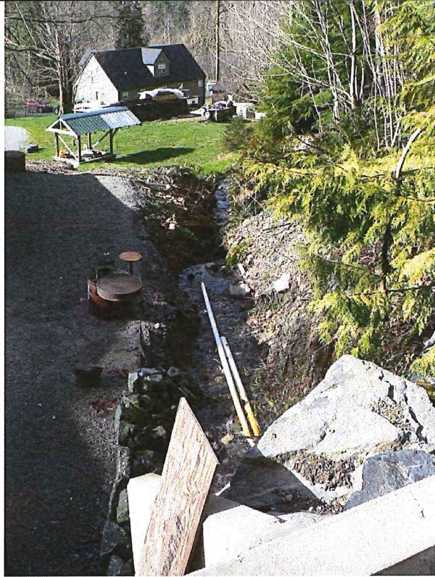
Photograph 4. View downstream from top of pipe outlet to ditchline.
