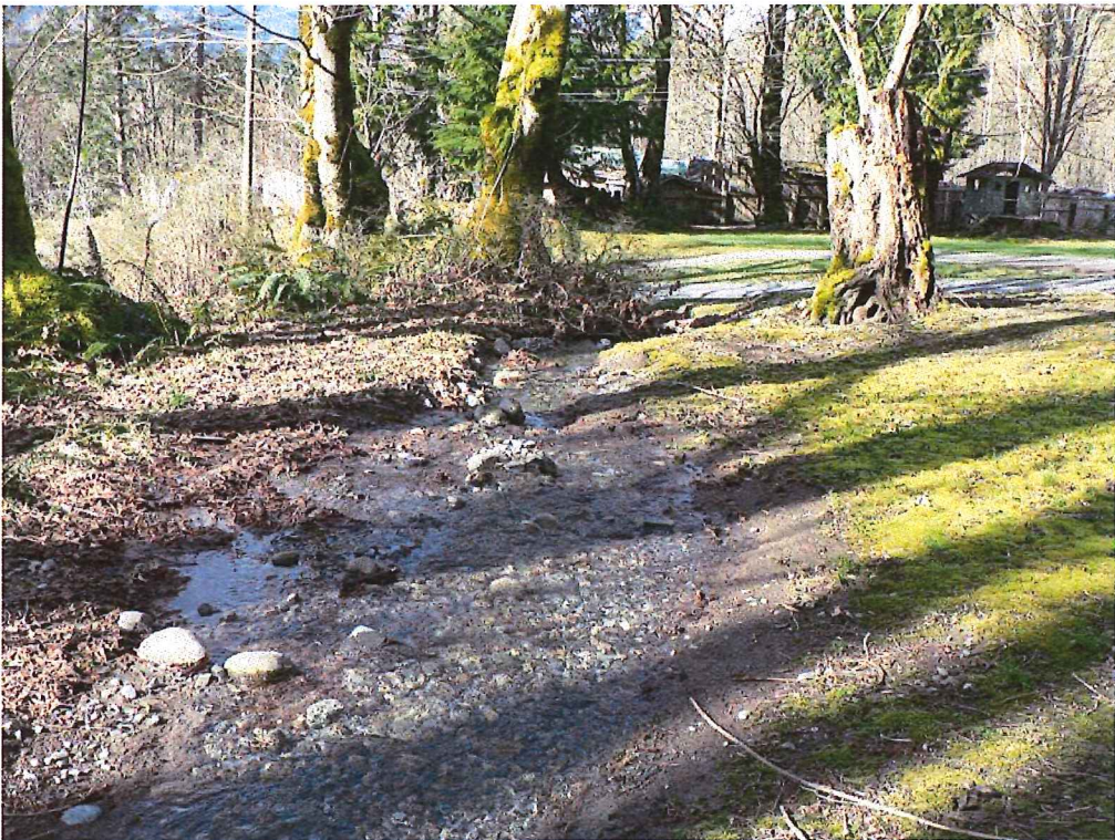
Photograph 9. View downstream on ditch drainage showing raised channel bed and lack of defined banks.
