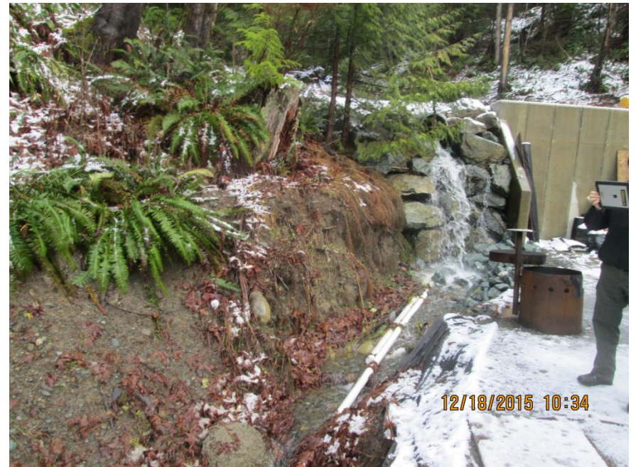
Armoured waterfall with concrete retaining wall looking north
