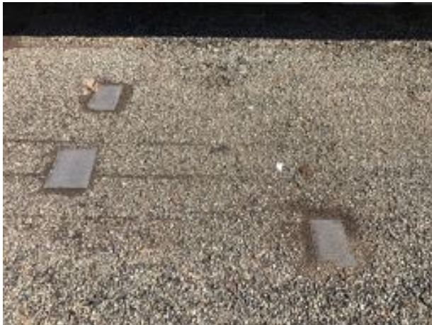
Photo 11 – Three additional repairs
