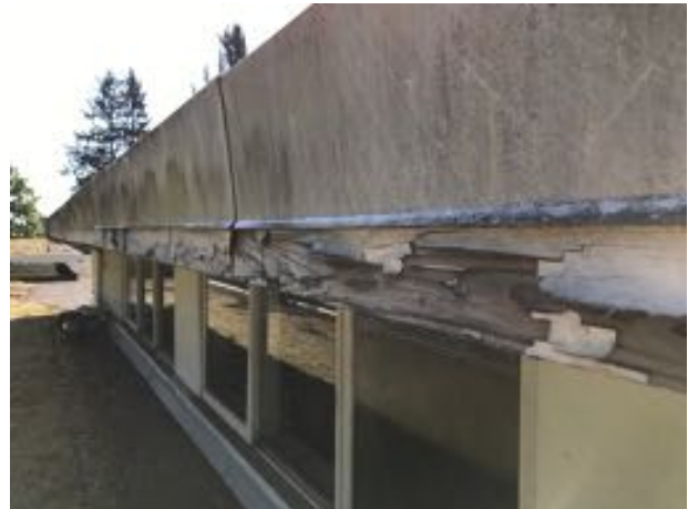
Photo 8 – Typical flashing and fascia boards
