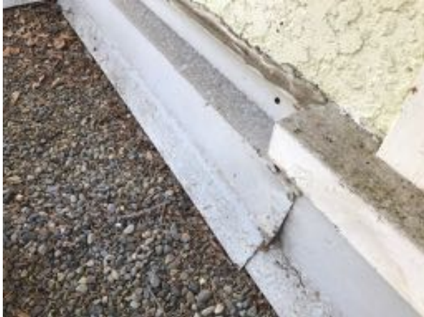
Photo 21 – View of base wall flashing and sealant at roof-to-wall interface
