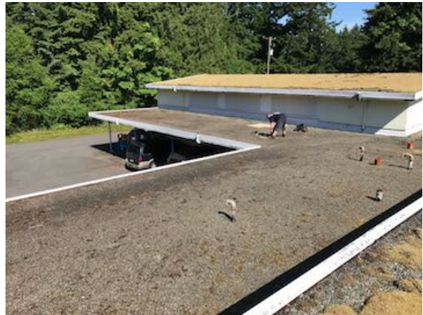
Photo 2 – An overview of Roof Type II
