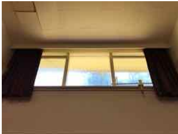
Photo 3 – Typical clerestory window
