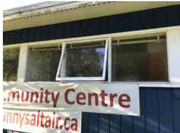
Photo 4 – Typical window at gymnasium kitchen
