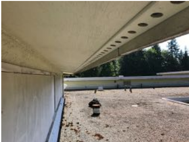
Photo 7 – Typical wood soffit with a vent strip
