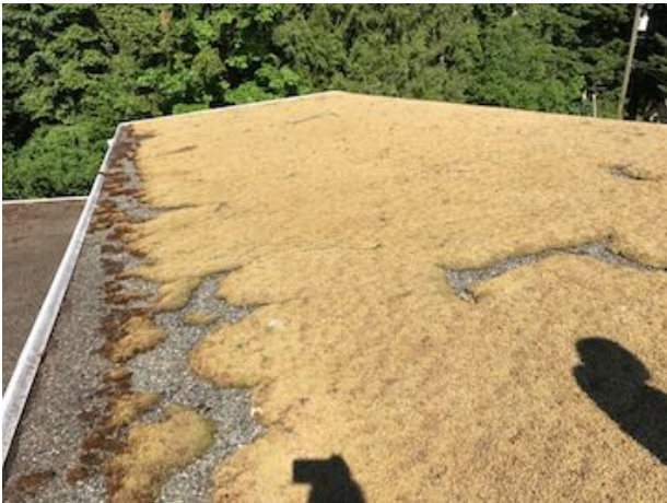
Photo 1 – An overview of Roof Type I
