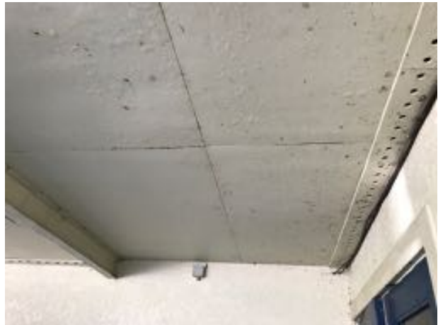
Photo 12 – Blistering paint finish and microbial growth on painted wood soffit
