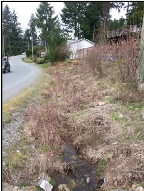
Looking north along the roadside ditch that runs parallel to Meadowview Road. Water is directed onto the subject property, from the roadside ditch via a CMP.
