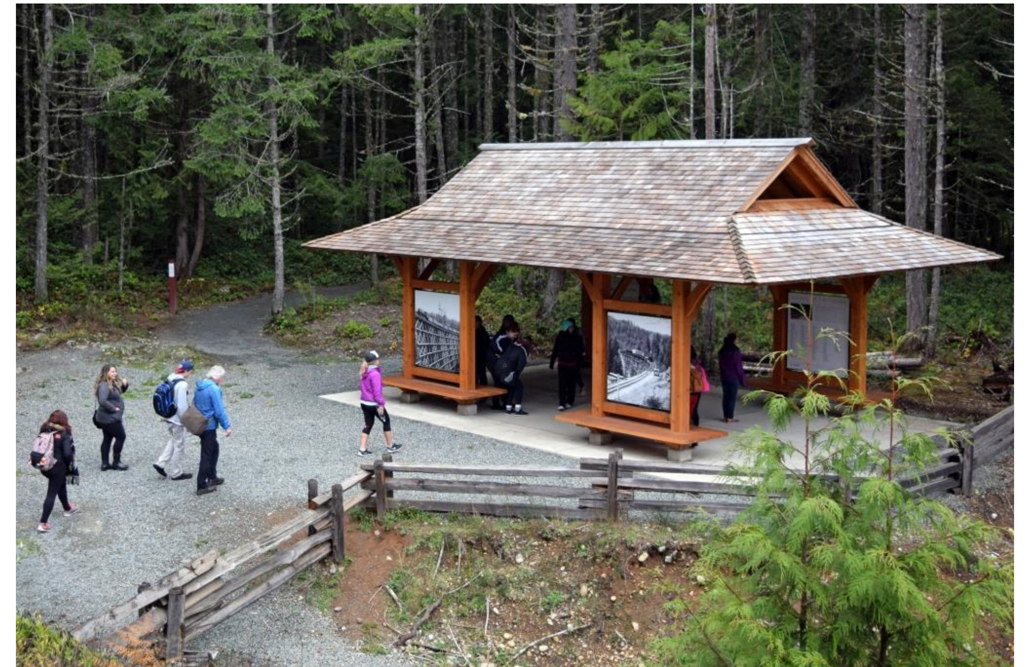
Kinsol Trestle Interpretive Kiosk
