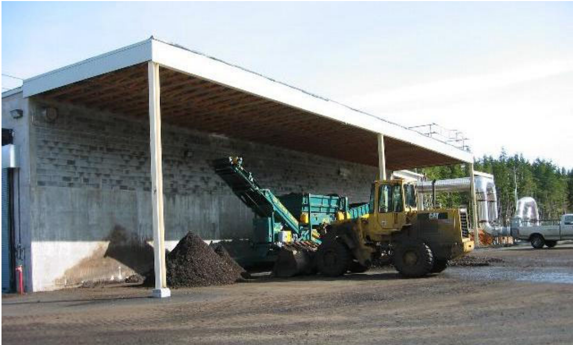
Screening Finished Compost Under cover on a Paved Pad
