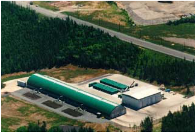
A Stinnes-Enerco In-vessel Composting Facility
