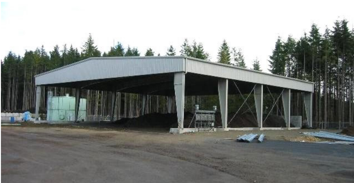
An Aerated Curing System Under Cover on a Paved Pad
