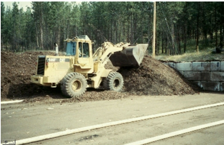
Building an Extended Aerated Static Pile Compost Pile at an Interior B.C. Facility
