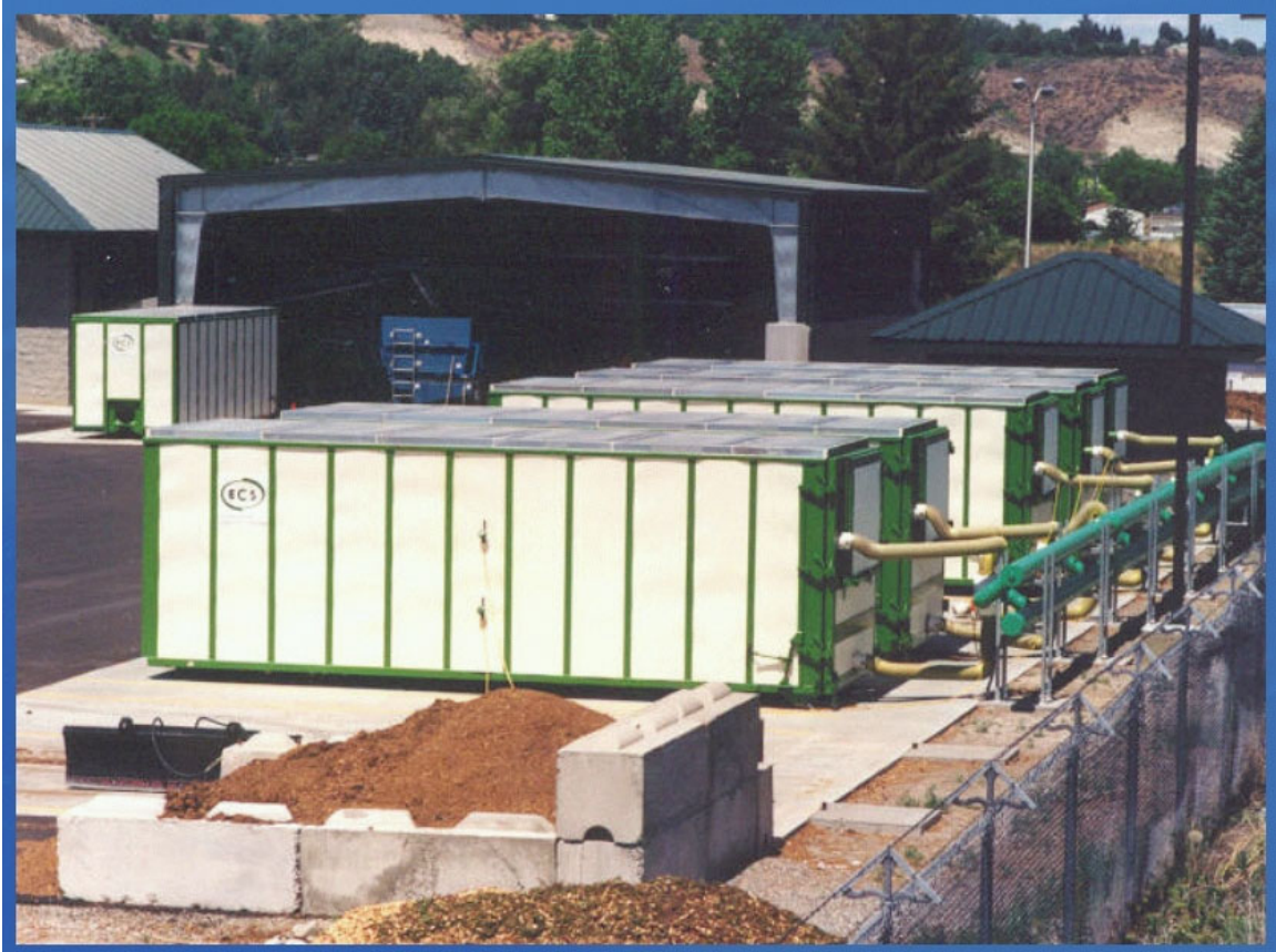
A Containerized In-vessel Composting Facility (courtesy of Engineered Compost Systems)
