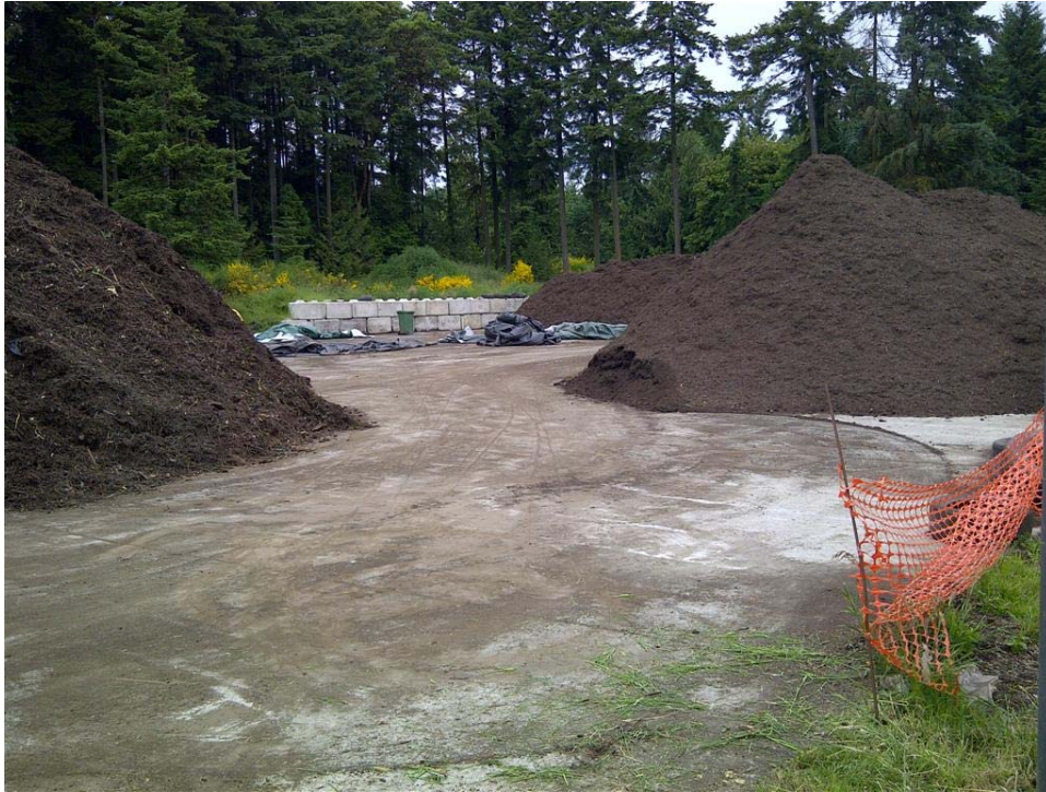
Photo 7: Piles in the screening area at the northwest corner of the site. Note concrete pad.
