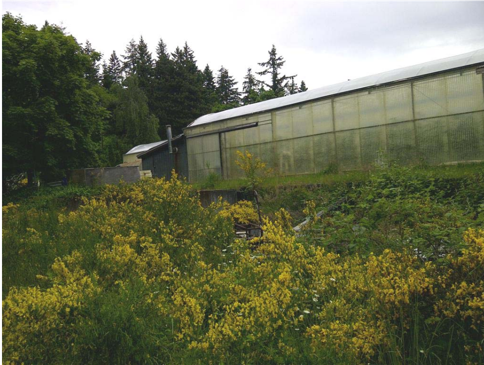
Photo 9: Looking at the exterior of the greenhouse building at 1375 Fairfield Road.
