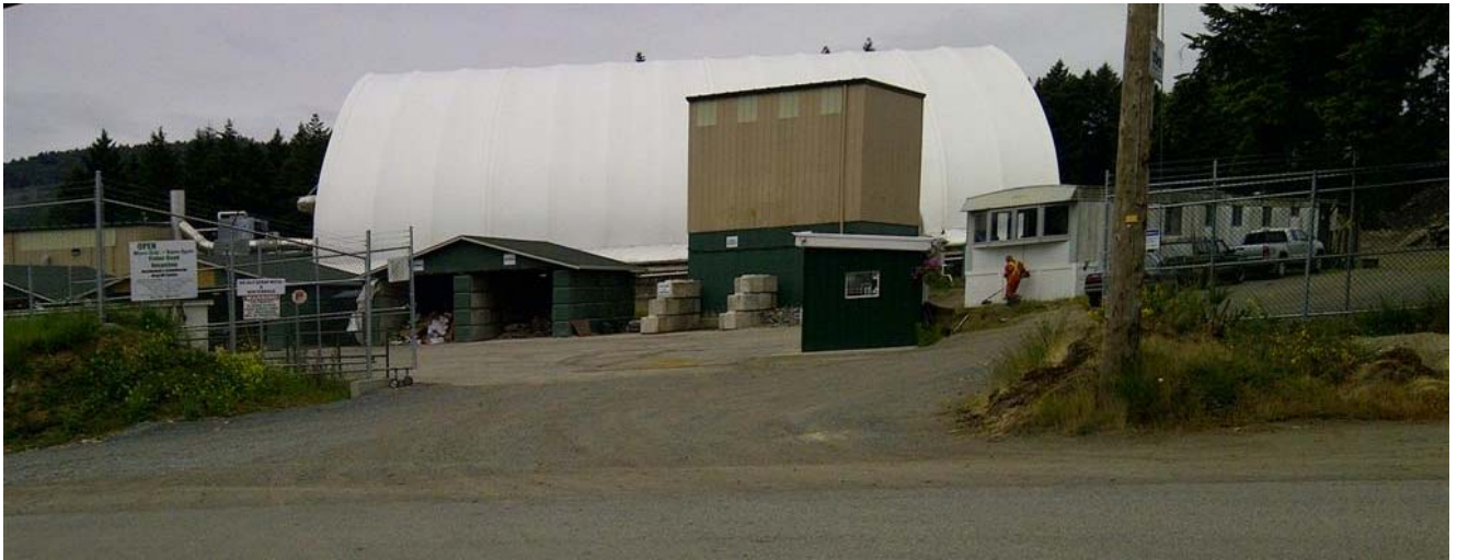
Photo 1: Looking northwest at the entrance from Fisher Road. The large white building is the compost receiving and processing building. The green buildings at left are storage bins for the recycling centre. The scale is in the foreground.
