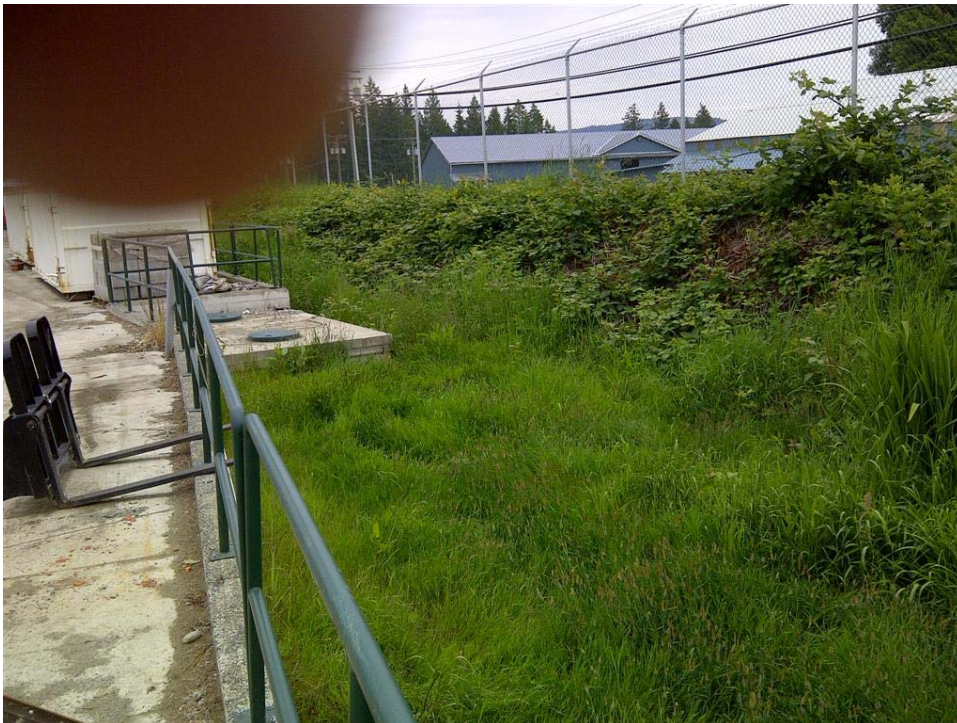
Photo 8: Swale area near the eastern property boundary. The edge of the recycling area pad is visible on the left with the oil/water separators visible at left.
