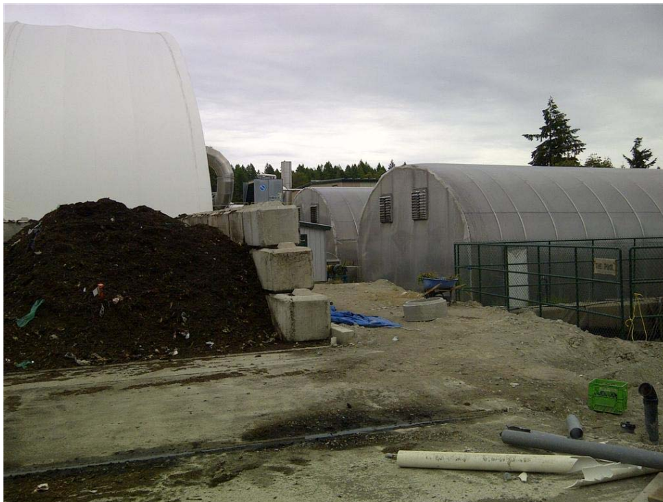
Photo 2: Looking southeast at the north end of two of the PVC covered bio-filter buildings (on right), with a portion of the south end of the outdoor curing pad air floor visible on the left and compost curing building behind. The fence on the right is for a leachate pond.
