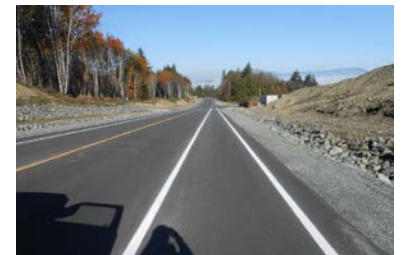
Roadside walkway – Sangster Road looking north
