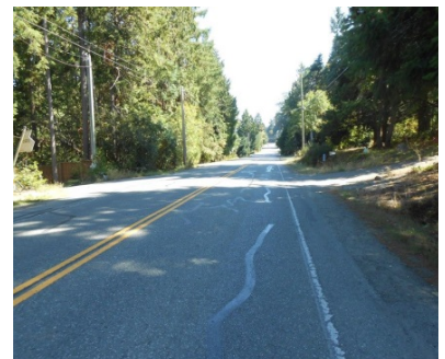
Mill Bay Road shoulder walkway
