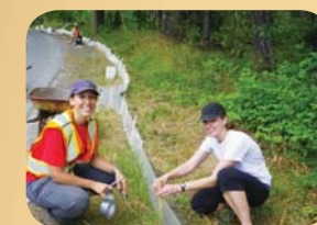
Volunteers installing drift fencing and pitfall traps to help move the toadlets across the road.
