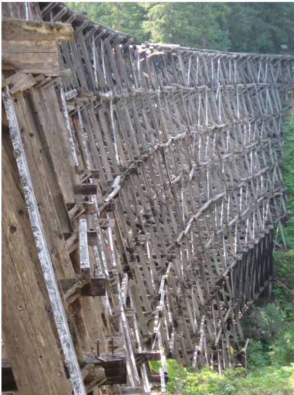
Kinsol Trestle prior to rehabilitation work beginning
