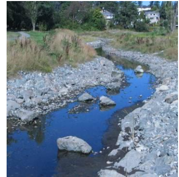
Stormwater infiltration swale
