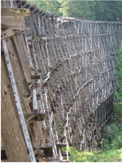
Kinsol Trestle View from North side
