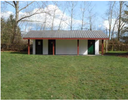
Coverdale Watson Park Washroom Building
