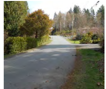
Shared Roadway – Pritchard Road
