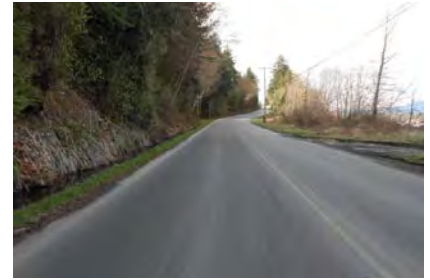
Cowichan Bay Road - section through the Theik Reserve land. Proposed Separated multi use pathway along foreshore.
