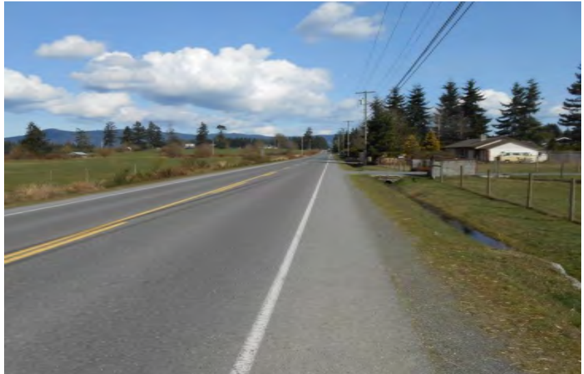
Roadside walkway – Koksilah Road looking east
