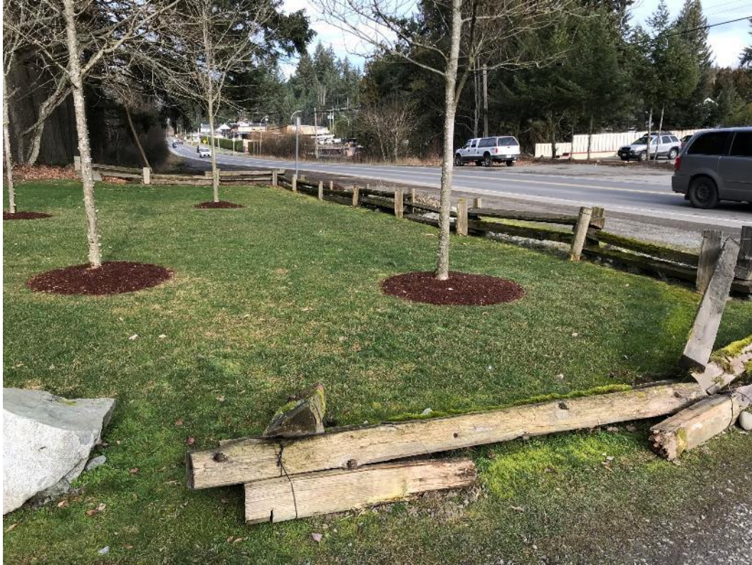
Split rail damaged from vehicle impact
