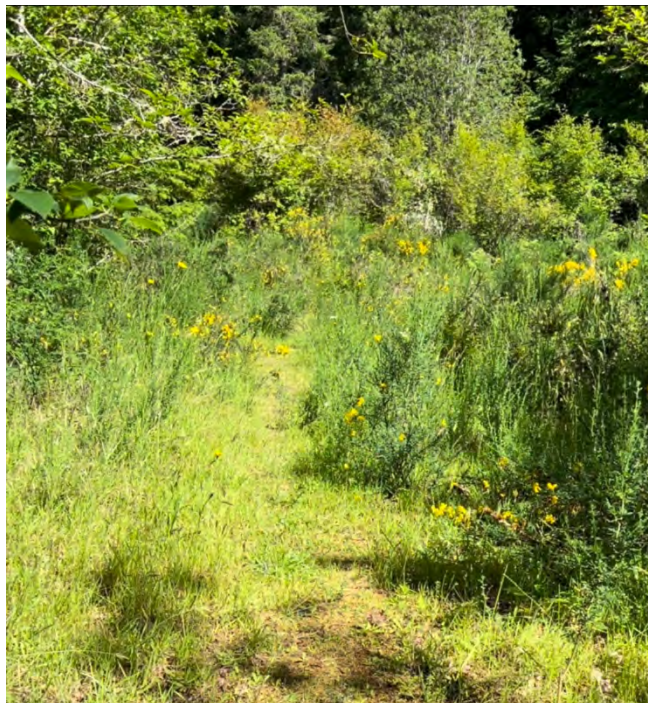
PHOTO 2. EXISTING ROAD OVERGROWN WITH SCOTCH BROOM
