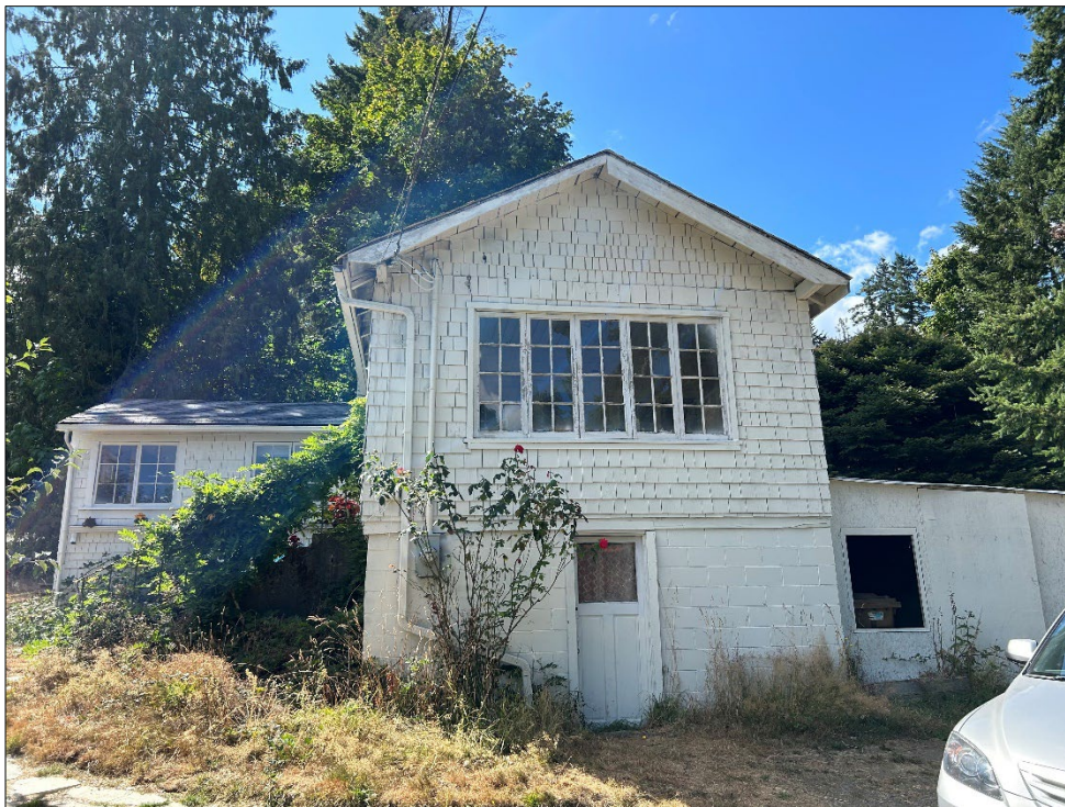
Photo from front yard, southeast corner of property. Existing dwelling (to be demolished), located on Proposed Lot 1.
