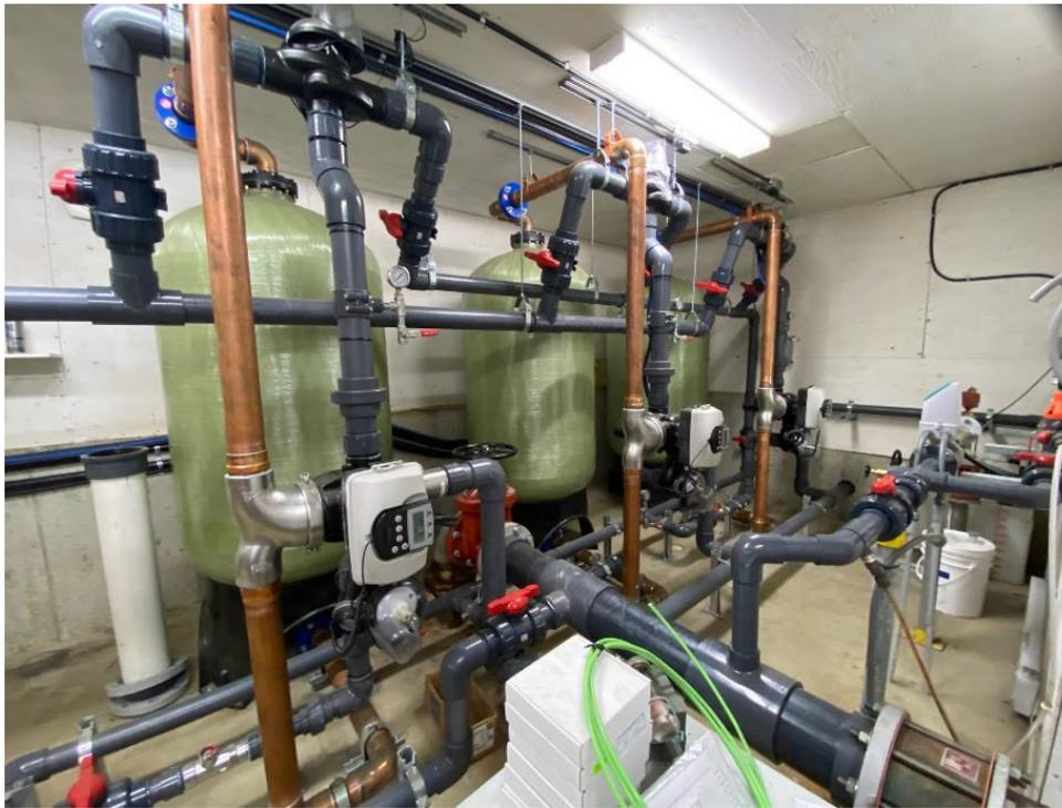
Backwash water during cleaning of the media filters
