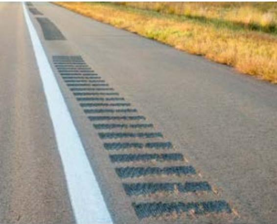
The BC Active Transportation Design Guide describes rumble strips as milled sections of the pavement along a roadway that provides feedback to motorists through noise and vibrations in the steering wheel, notifying them when they have deviated from the travel lane into the shoulder. Rumble strips are intended to clearly delineate the shoulder area and ensure the additional road width does not lead to higher vehicle operating speeds.
