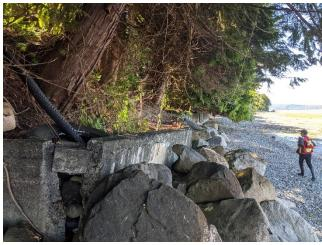
Photo 025: Retaining wall failure and toe of slope bulging.
