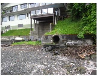
Photo 012: Stormwater outfall.
