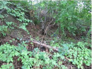
Photo 004: Suspected shallow surficial failure along unprotected shoreline segment. One-metre-high scarp at base of slope along shoreline comprised of suspected colluvium (loose, silty sand with pebble to cobble inclusions).
