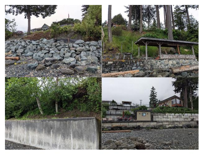
Figure 6. Example erosion mitigation observed along the study area shoreline.
