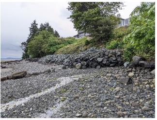
Photo 007: Stream outlet. Recent riprap installation at the toe of the slope/upper beach face. Adjacent natural segments of shoreline are actively eroding till.
