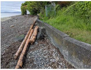
Photo 019: Retaining wall failure and slope bulging at toe.
