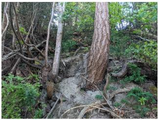
Photo 028: Failure on 39-degree slope. Upper portions of the slope near vertical. Downed tree and rootball exposed.
