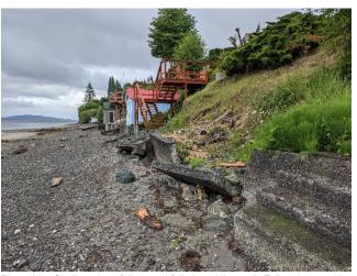
Photo 017: Shallow slope failure and failed retaining wall. Failure is approximately 7 m wide and 0.5 m deep on 32-degree slope.
