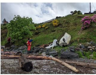
Photo 018: Shallow failure on 45-degree slope.
