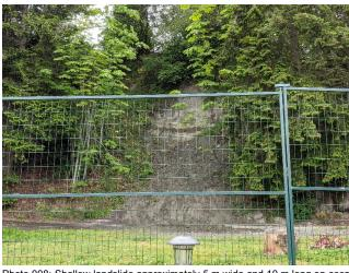
Photo 008: Shallow landslide approximately 5 m wide and 10 m long on escarpment backing property.
