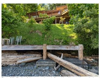
Photo 029: Shallow failure approximately 5 m wide with up to 1 m vertical displacement.
