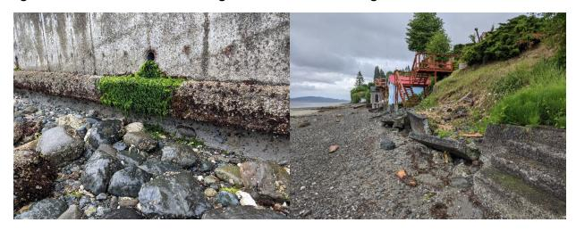
Figure 8. Observed undercutting of a seawall within the study area with consolidated till visible below concrete footing (left). Shallow landslide and failed retaining wall/seawall (right).
