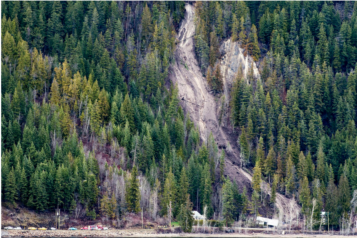
Image 1: Development at the toe-of-slope faces increased risk.
