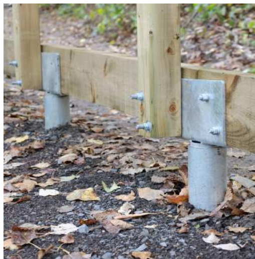
..... Left: Helical pile foundation .....
