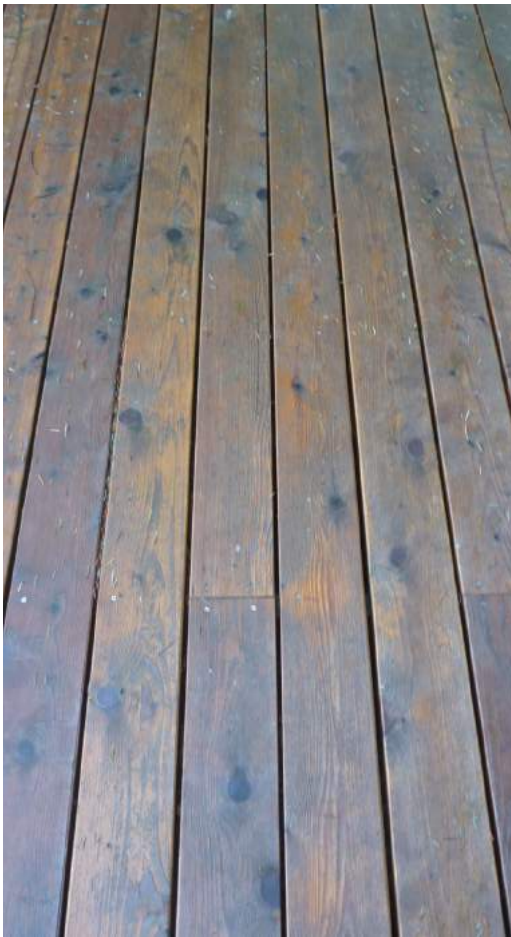
Decking nailing pattern
